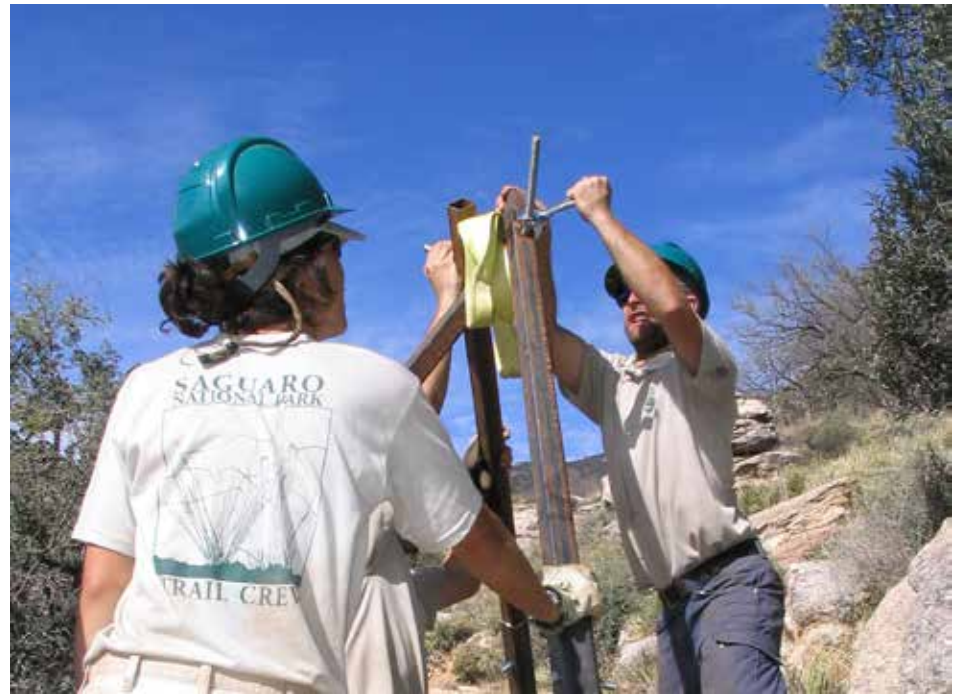
Trails in Saguaro National Park are maintained by our Trail Crew, and projects are funded from fee dollars. Here the crew is rigging equipment to move large rocks out of the trail.
