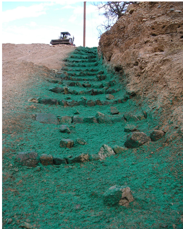
Rock step terrace with hydromulch and seed.
