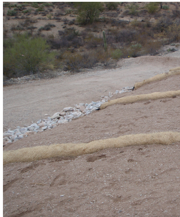
Wattles used to slow and retain water, prevent erosion, and stabilize soil to promote plant establishment.
