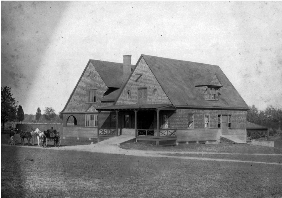
Figure 3. View looking northeast at the west facade of the stable and lodge, 1905. The carriage road/service road provided access to the building (SAHI, #1112, Box 6).
