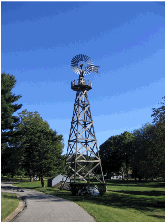
Figure 27. View looking north at the windmill and pump house (OCLP, 9-22-05 142, 2005).
