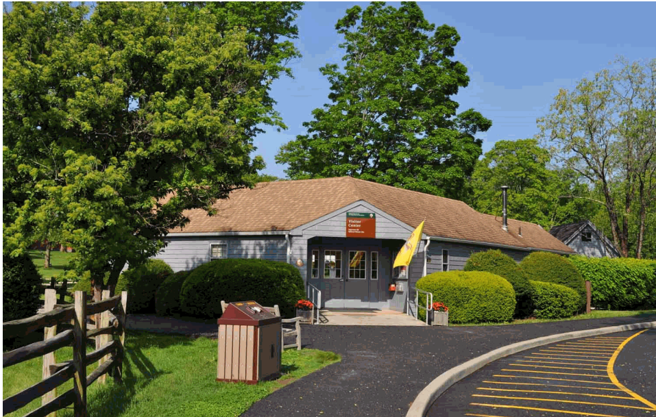
Figure 28. View looking northwest at the visitor center (OCLP, DSC_0355, 2012).
