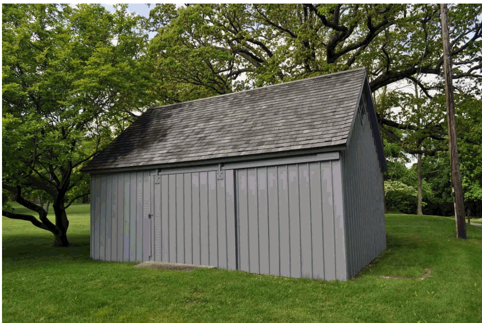
Figure 25. View looking west at the gardener's shed (OCLP, DSC_0513, 2012).
