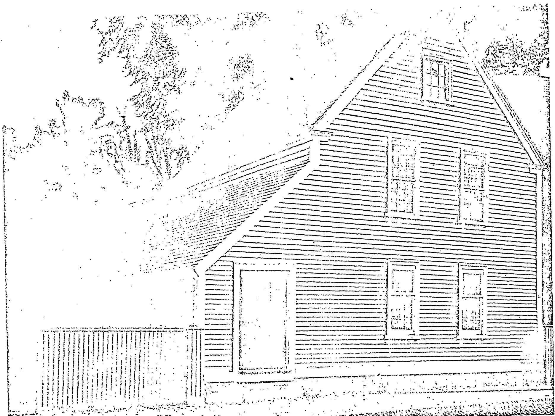
Fig. 7. Leantos and street gable end, from the original Wilfred A. French. negative (no. 24254). exposed about 1924 to 1927. Courtesy for the
