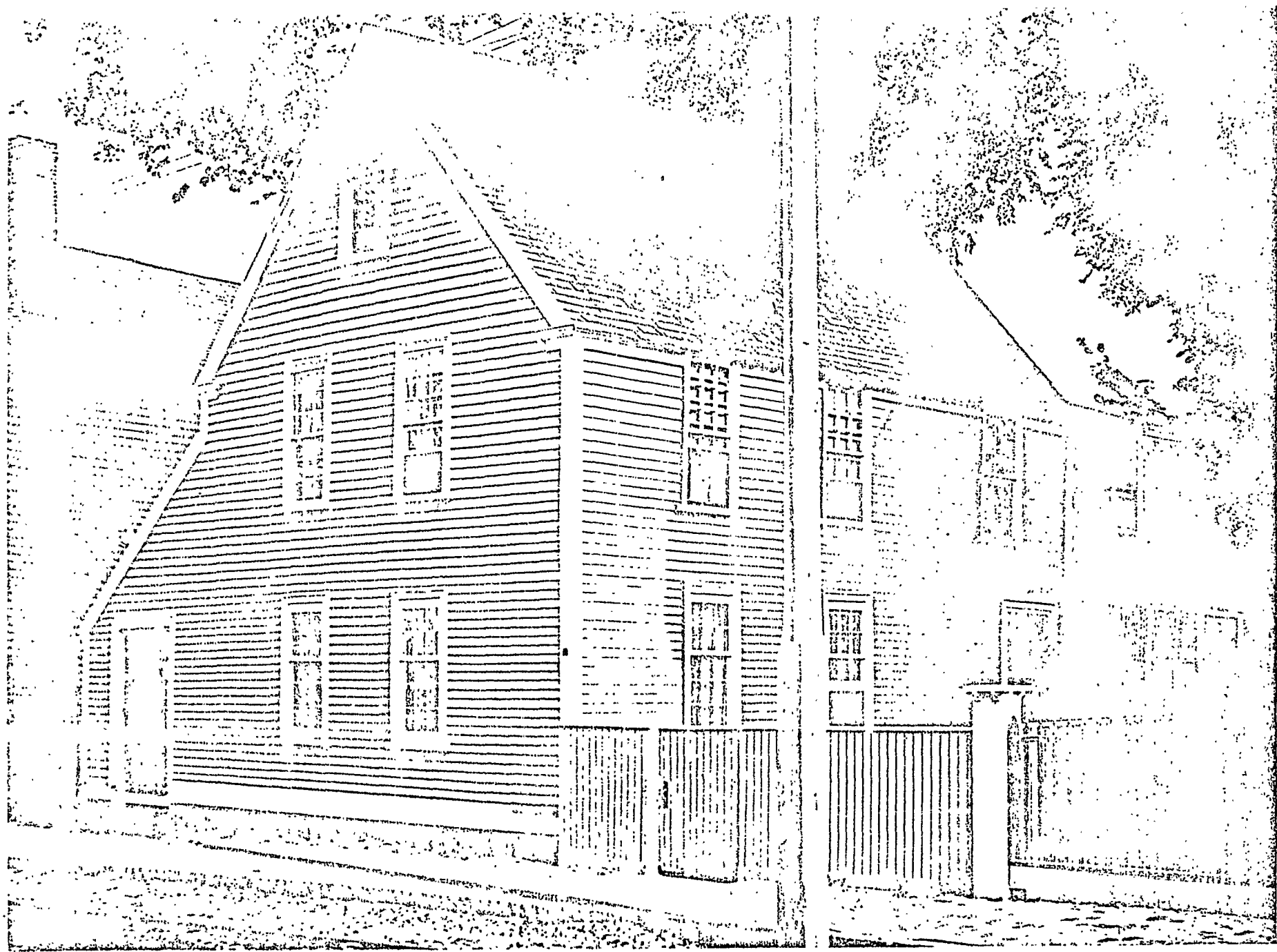
Fig. 11. West front and street gable end, from the original Wilfred A. French negative (no. 2908B), exposed about 1884 to 1895. Society
