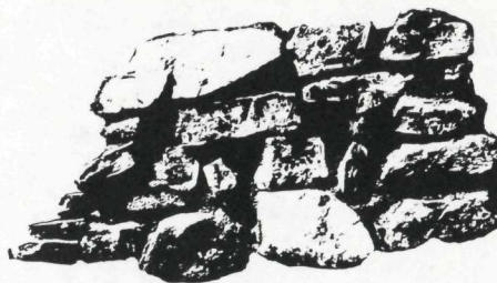
Masonry construction represents the final building development at Gran Quivira. Limestone was easily obtained, for it underlies the entire area. The mortar consisted of a sandy material mixed with earth, ashes, and fibers. Today the ruins are stabilized.
