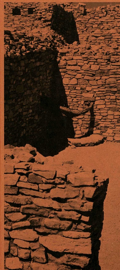
This room was the friar's quarters. The curved log set into the walls supported the hood above the fire.
