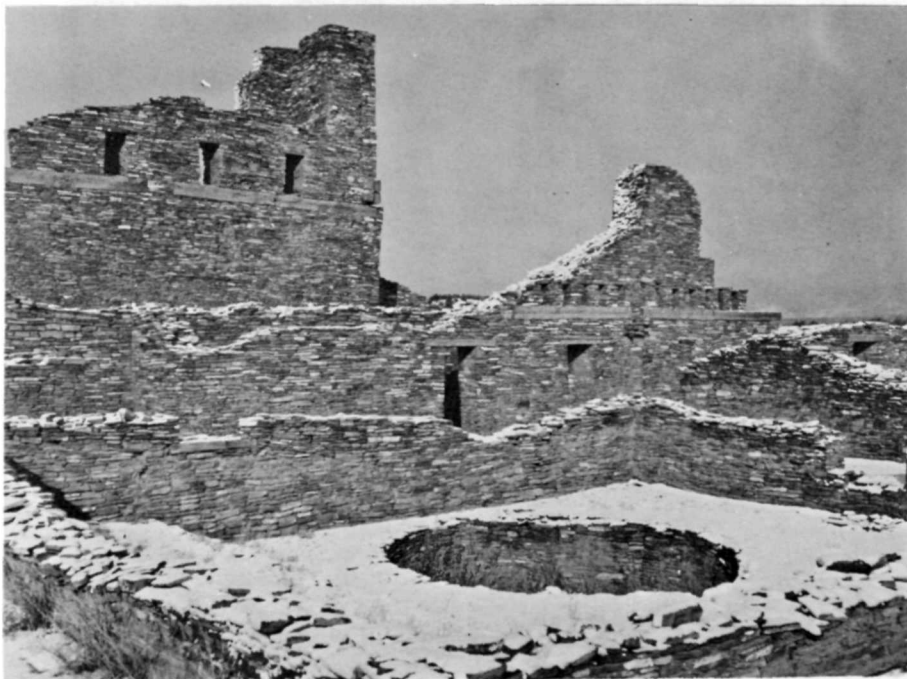
Part of Abo church and convento ruins, circular Indian kiva in patio
