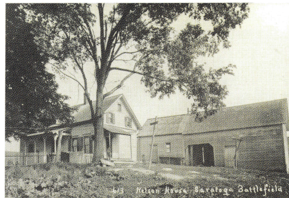
Neilson House and outbuildings ca. 1920
