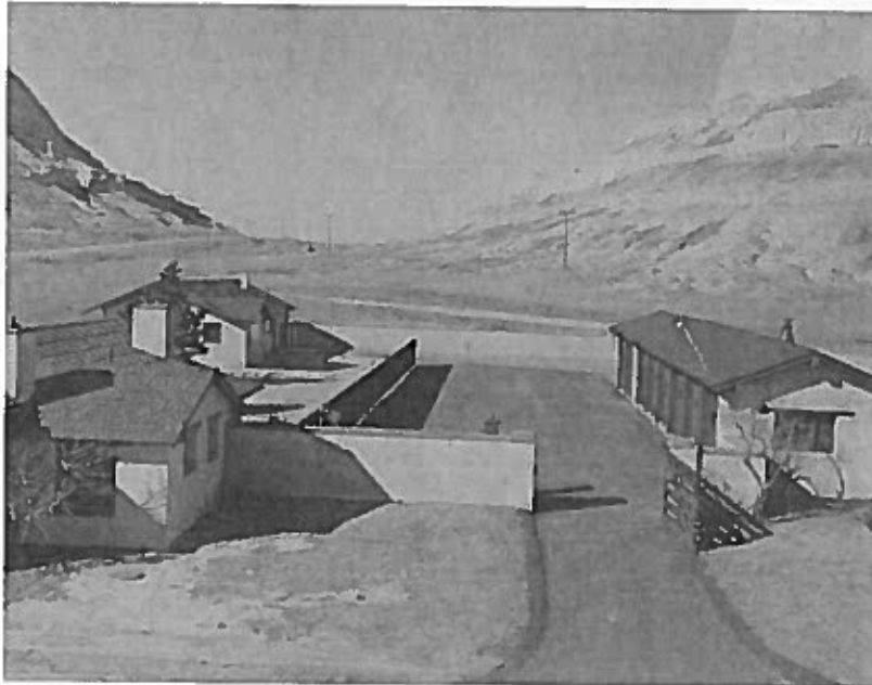
Figure 38. Maintenance Shed, Ranger's Residence, Mission 66 Residence, and courtyard, c. 1958. Image courtesy of Scotts Bluff National Monument.
