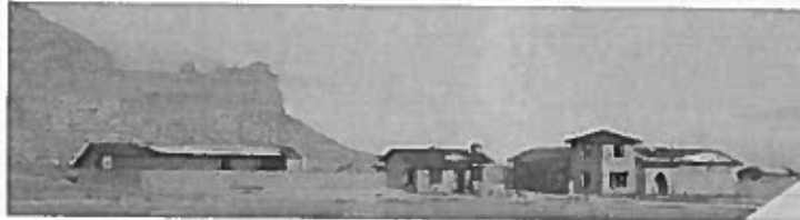
Figure 26. Visitors Center complex, c. 1939. Image courtesy of Scotts Bluff National Monument.
