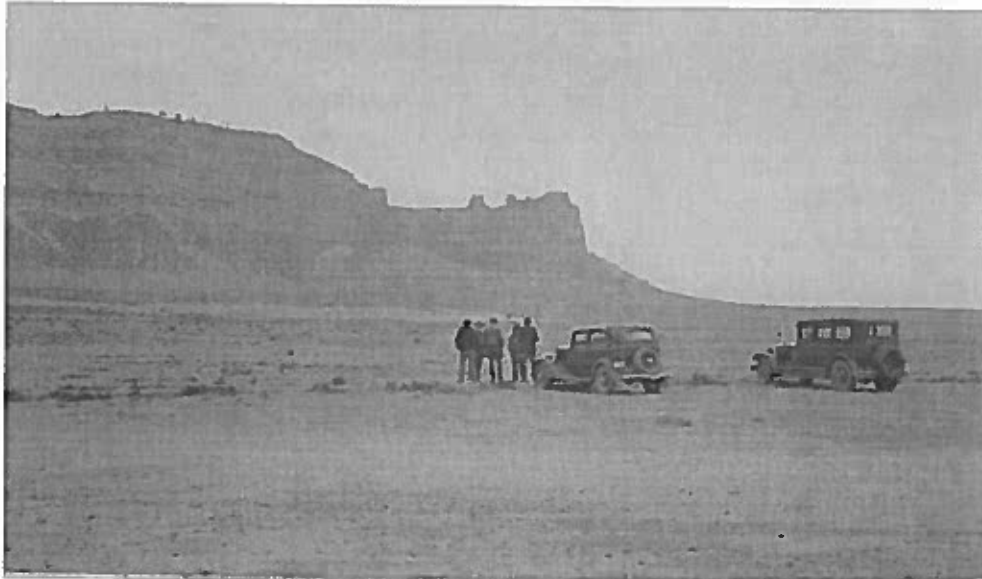
Figure 16. From left to right: Sam Serano, Charles Randals, Howard Baker, and Harold Cook survey the future site of the Visitors Center at the base of Scotts Bluff, February 20, 1935. Photo by F. H. Shoemaker, courtesy of Scotts Bluff National Monument.
