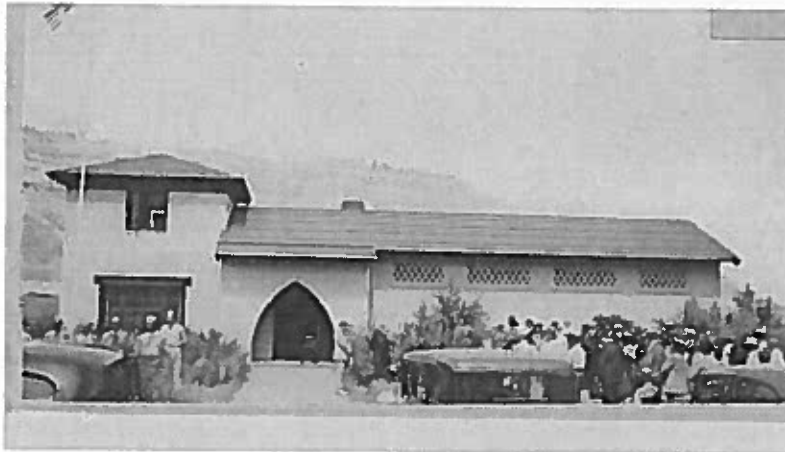
Figure 27. Visitors Center, c. 1942. Image courtesy of Scotts Bluff National Monument.
