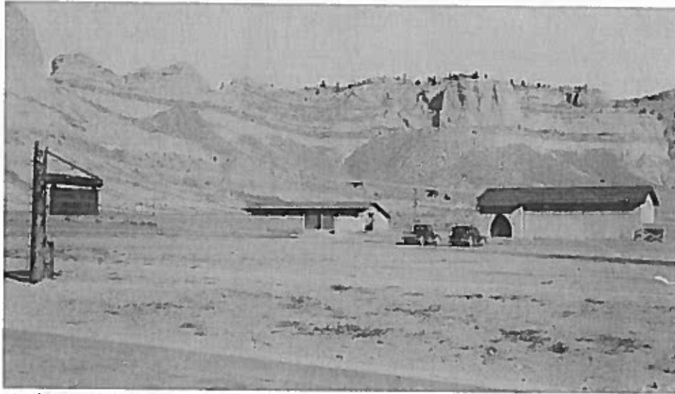
Figure 21. Maintenance Shed and Visitors Center, c. 1937. Image courtesy of Scotts Bluff National Monument.
