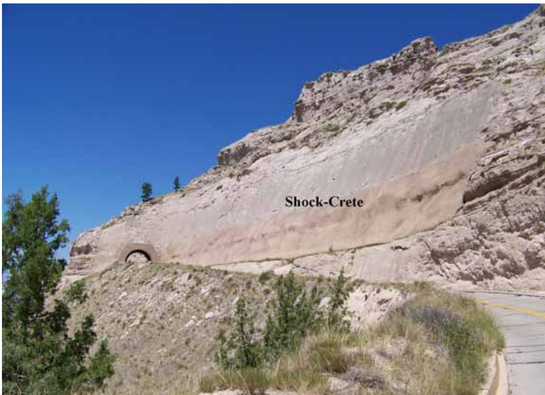
Figure 6. Shot-crete (shock-crete) helps to stabilize the slope between tunnels 2 and 3 on Summit Road in Scotts Bluff National Monument. Photograph by John Graham (Colorado State University), July 7, 2007.
