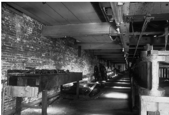
Lowell National Historical Park, Massachusetts. National Park Service photo.
