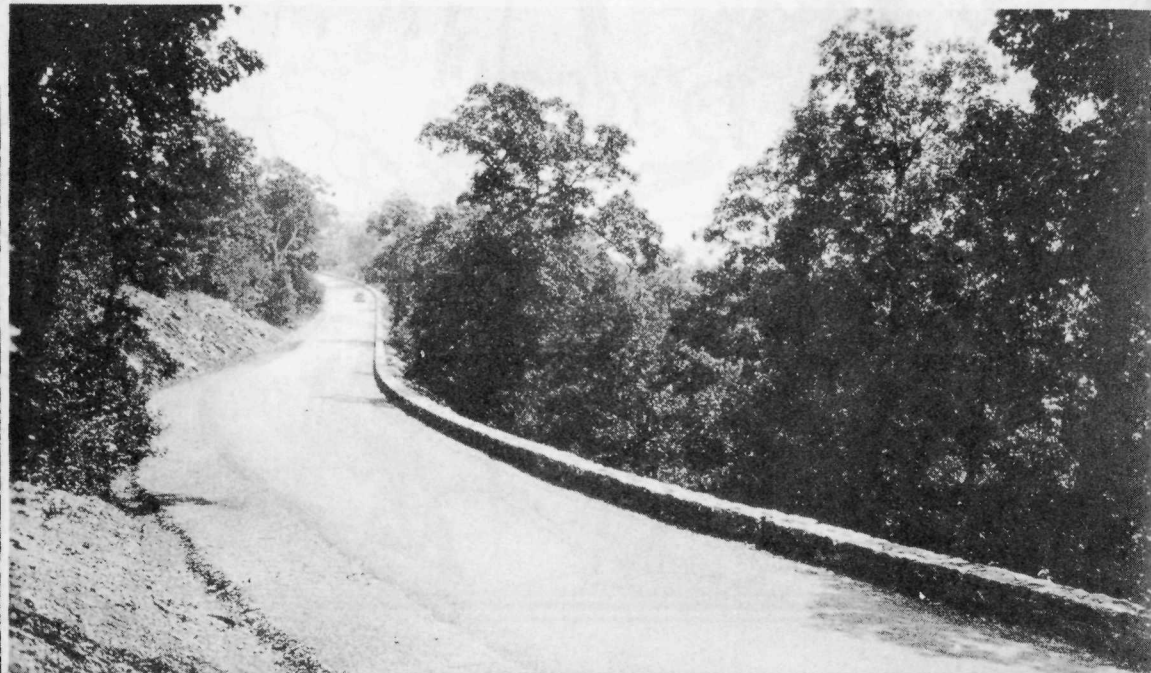
A VIEW OF THE SKYLINE DRIVE, SHOWING PROTECTIVE STONE GUARD WALL ERECTED ALONG STEEP FILL.
