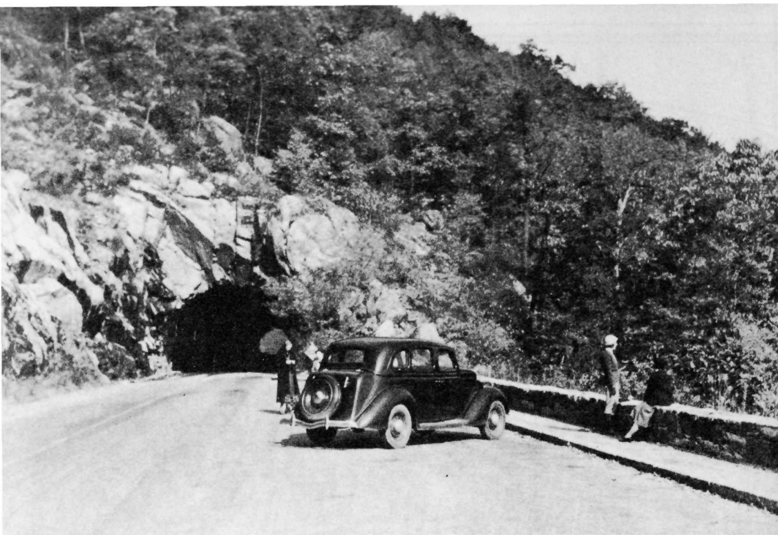
SOUTH PORTAL OF THE 700-FOOT TUNNEL THROUGH MARY'S ROCK, NEAR PANORAMA. BORED THROUGH SOLID GRANITE, IT IS ONE OF THE OUTSTANDING ENGINEERING ACCOMPLISHMENTS IN THE CONSTRUCTION OF THE DRIVE. Virginia State Chamber of Commerce Photo
