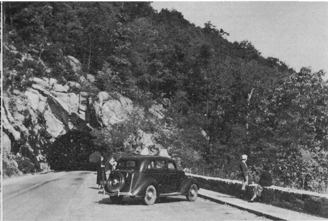
THIS IS THE SOUTH PORTAL OF THE TUNNEL ON SKYLINE DRIVE JUST SOUTH OF THORNTON GAP. IT IS BORED 700 FEET THROUGH THE SOLID GRANITE OF MARY'S ROCK AND IS ONE OF THE OUTSTANDING ENGINEERING ACCOMPLISHMENTS IN THE CONSTRUCTION OF THE HIGHWAY. Virginia State Chamber of Commerce Photo
