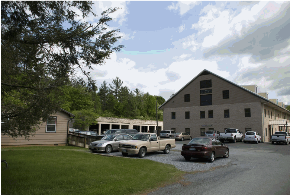
Figure 21. View of the Maintenance Building constructed in 1995 with the Equipment Storage/Workshop beyond (OCLP, 2008).
