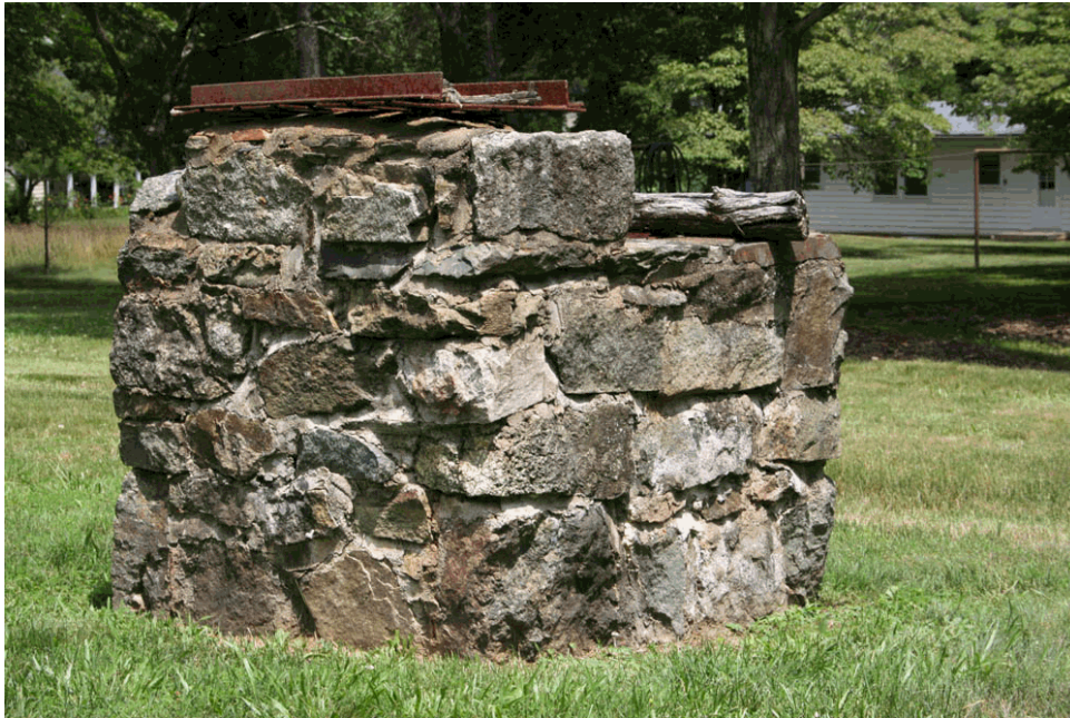
Figure 24. View of one of two stacked stone grills located in the residential area at Headquarters (OCLP, 2008).
