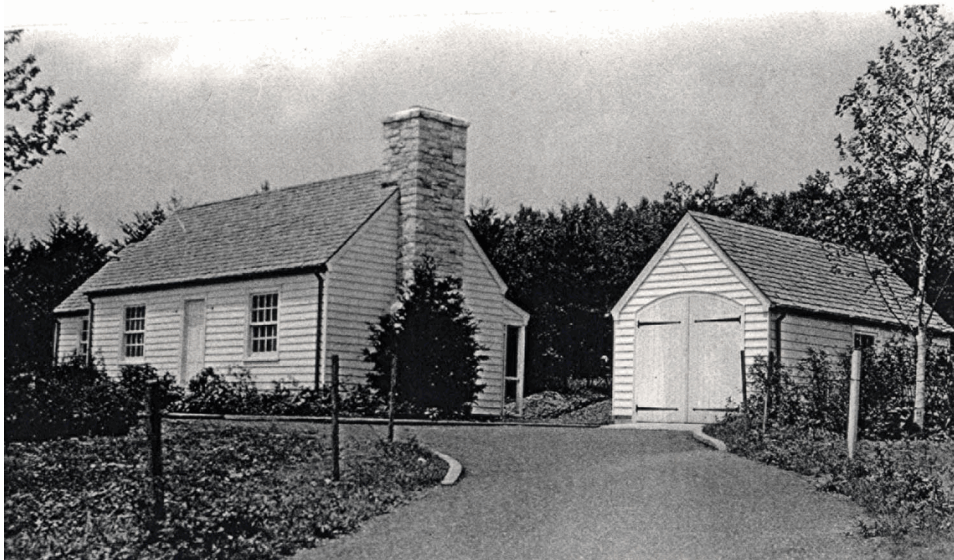
Figure 8. View of one of the employee residences constructed at the Headquarters site in 1941 (Shenandoah NP Archives, Negative No. 627-5). Note the variety of shrubs and trees planted, including a newly staked tree to the right.
