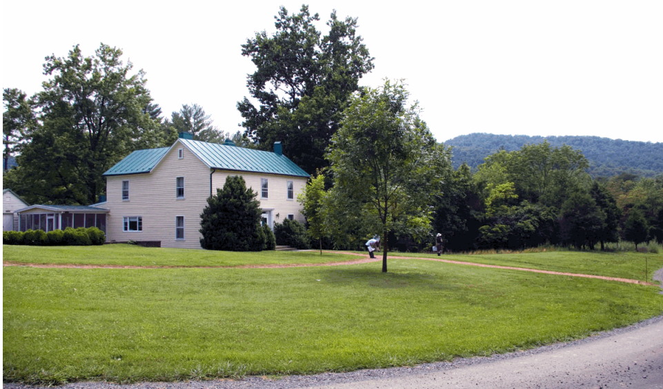
Figure 17. View of open lawn at the former Superintendent's Residence (OCLP, 2008).
