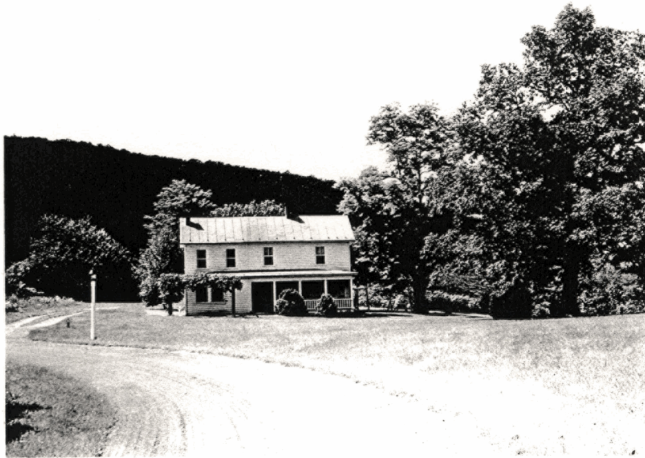
Figure 9. View of 1916 farmhouse used as a residence, one of two pre-existing park buildings at the Headquarters site (Shenandoah NP Archives Negative No. 627-30B). Note the wooden lightpost to the left along the access road.
