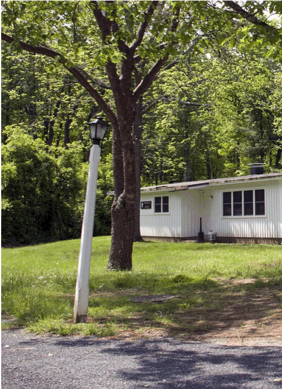
Figure 23. View of one of seven original wood lamp posts in the residential area of the Headquarters site (OCLP, 2008).
