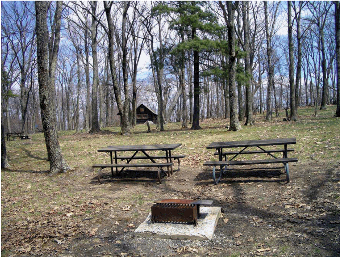
Picnic Grounds with the Picnic Area Comfort Station in the background, looking east (OCLP, 2005).
