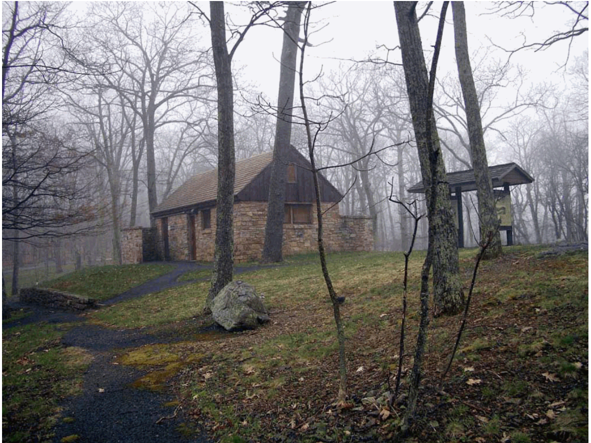
Campground Comfort Station, Campground Comfort Station Retaining Wall and Camp Ground Information Kiosk (OCLP, 2005).
