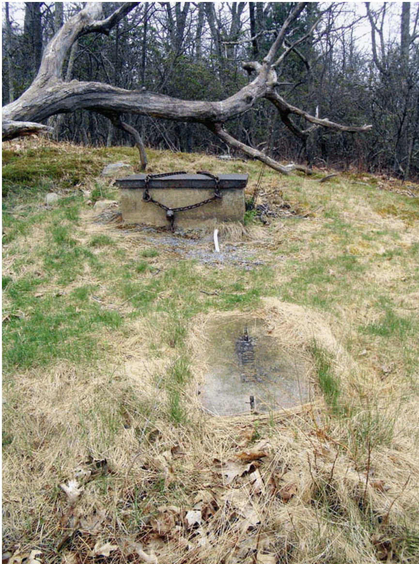
Water Reservoir on hillside above Campground, looking northeast (OCLP, 2005).
