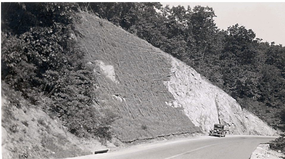
Figure 3. View of cribbing with chestnut logs to stabilize slope, early 1930s (SHEN website, image 20060706160746).
