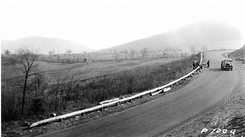
Figure 6. View of log guardrails installed by the CCC along Skyline Drive, early 1930s (SHEN website, image 20060706161152).
