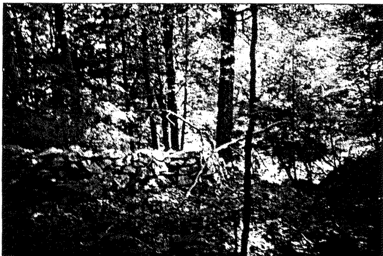
35. View east along the former Old Skyland Road roadbed showing the Gardens' perimeter stone wall, 1990
