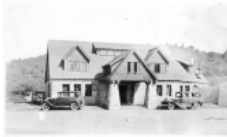
Located near the present day Panorama Restaurant, the Tea Room was the last remnant of resort. Virginia Sky-Line Company continued to serve park visitors in this facility until construction of the Highway 211 overpass necessitated its removal in the late 1950s. Photo courtesy of Shenandoah National Park Archives.
