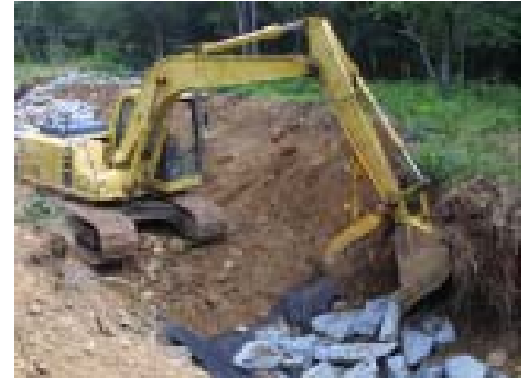
Excavator with thumb is essential for proper rock placement.
