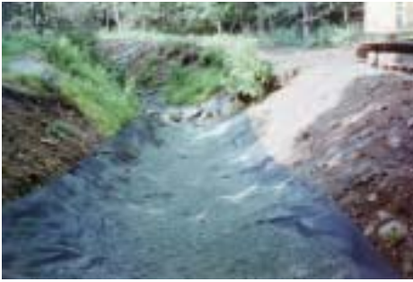
Geo-textile filter fabric secured with gravel.
