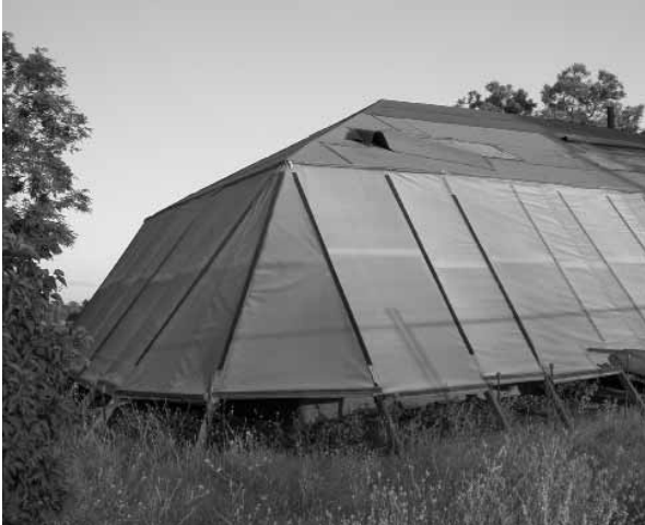
The Gil Adobe with protective tarps, NPS photo
