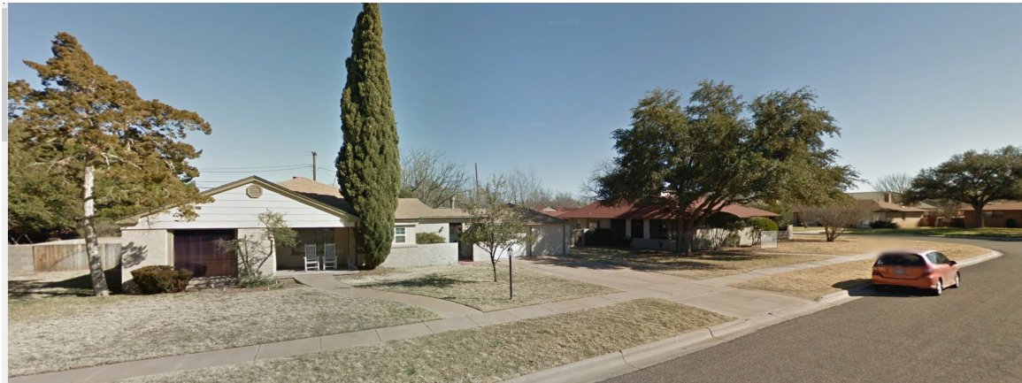
Figure 32. View of 402 East Broadway Street and Residence at 400 East Broadway Street, Looking Southeast Down Broadway Toward Ohio Avenue (Google Maps)
