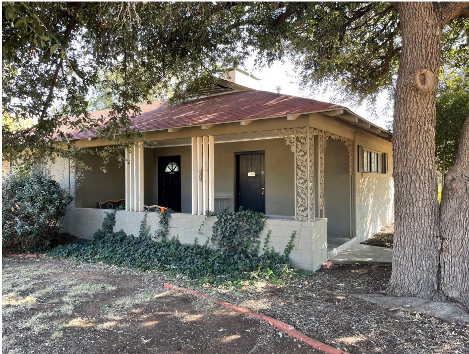
Figure 29. Staff Entrance to 400 East Broadway Street, Looking Southwest from Broadway Street (photo from THC Phase II Report, April 2022)
