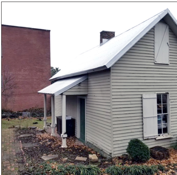
Figure 18. Garden Cottage (NPS Study Team 2019)
