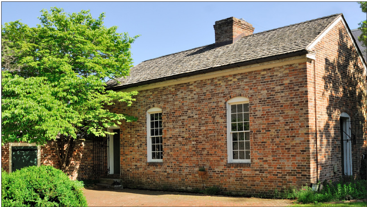
Figure 10. Reconstructed Kitchen (NPS 2014)
