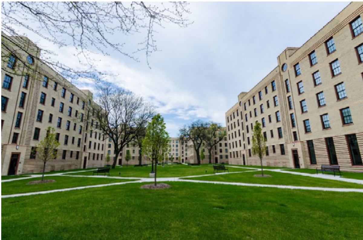
FIGURE 7. RESTORED ROSENWALD COURT APARTMENTS INTERIOR COURTYARD, 2017 (PHOTO BY ERIC ALLIX ROGERS, COURTESY OF OPEN HOUSE CHICAGO)
