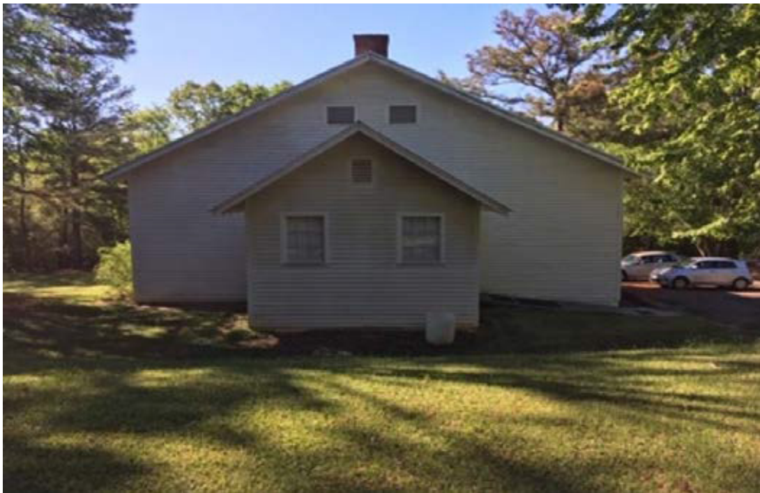
FIGURE 19. NOBLE HILL SCHOOL REAR ELEVATION, 2019 (DON STEVENSON) (EHT TRACERIES 2021A, 54, FIG. 49)
