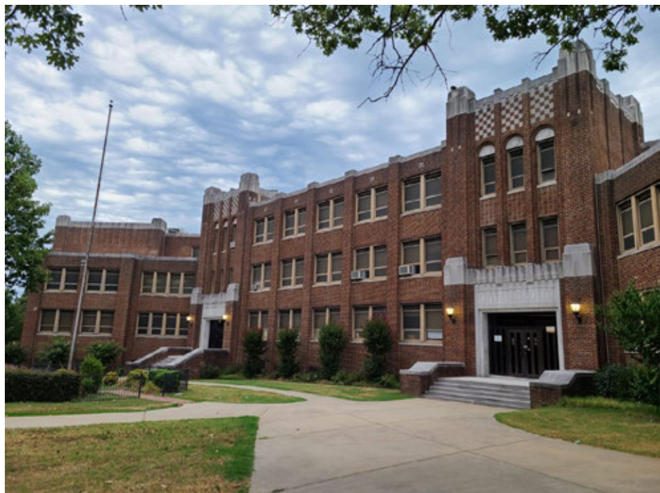
FIGURE 36. DUNBAR JUNIOR HIGH, SENIOR HIGH AND JUNIOR COLLEGE SOUTHEAST ELEVATION AND FRONT ENTRANCE, 2022 (PHOTO BY NPS STUDY TEAM)
