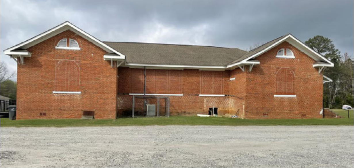
FIGURE 34. REAR VIEW OF ELMORE COUNTY TRAINING SCHOOL, 2023
