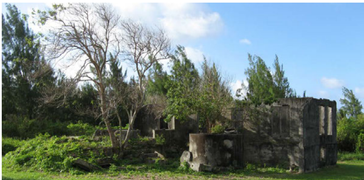
Tatachog rectory, constructed during the Japanese period on Rota. Photo: NPS.
