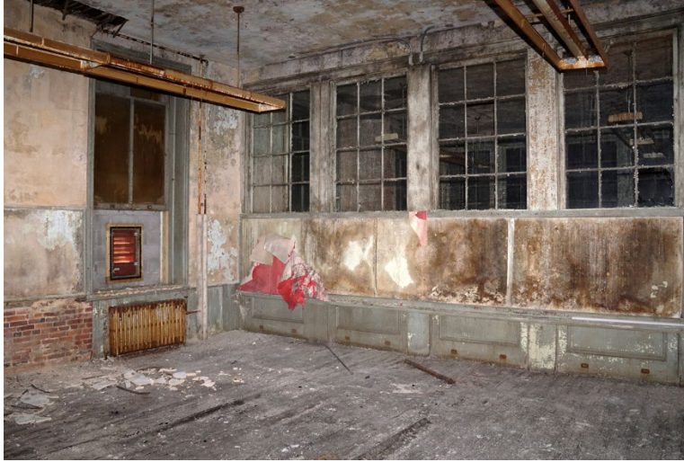
FIGURE 15. HISTORIC WINDOWED PARTITION IN A FIRST-FLOOR CLASSROOM (GLASSMAN 2019)
