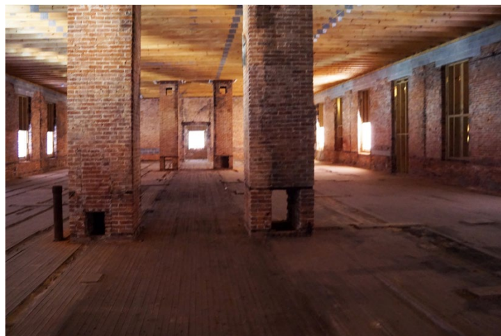
FIGURE 17. GUTTED SECOND-FLOOR VIEW DOWN THE HALLWAY (GLASSMAN 2019)
