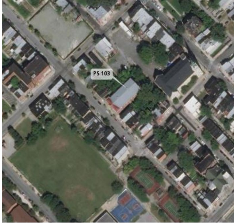
FIGURE 2. AERIAL VIEW OF P.S. 103 (MAXAR 2020)
