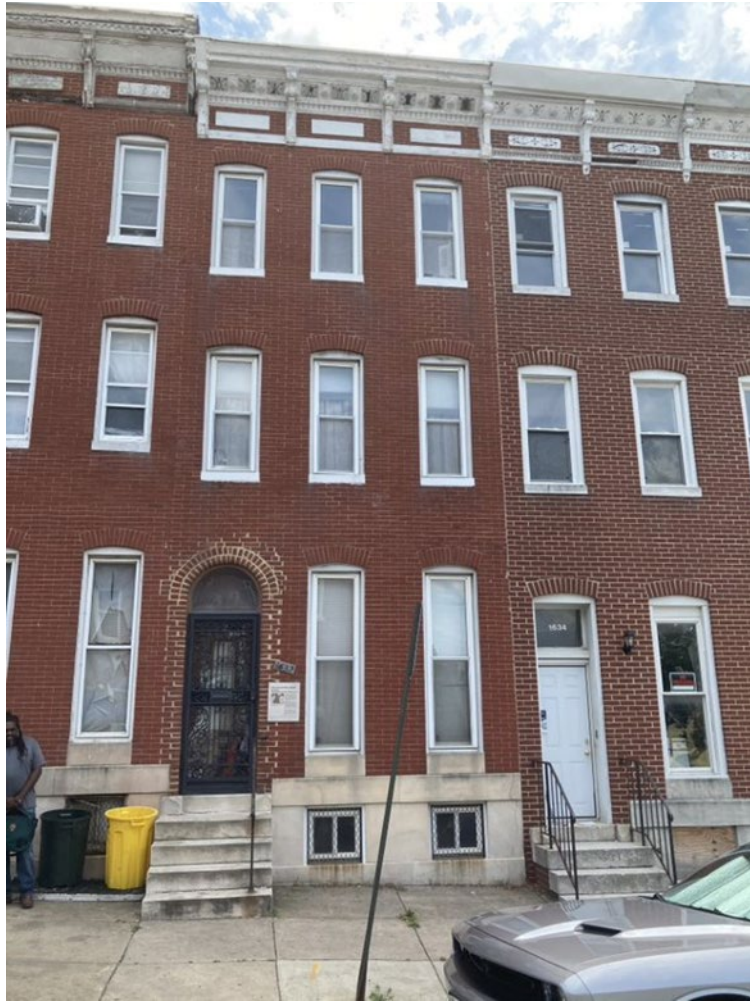
FIGURE 19. 1632 DIVISION STREET (CENTER), SHOWING ROW HOUSE CONTEXT, MARBLE STEPS, THREE WINDOW-BAY FAÇADE, AND ITALIANATE DETAILING (DROGE 2021)
