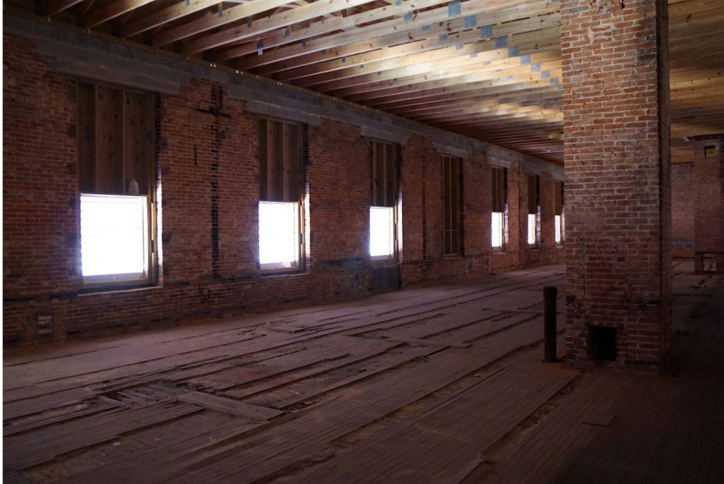
FIGURE 18. SECOND-FLOOR VIEW OF CLASSROOM. NOTE ORIGINAL FLOORBOARDS AND NEW ROOF (GLASSMAN 2019)
