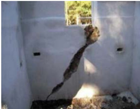
Cabin E14 showing a large crack in the front left wall, top left and bottom left. The picture on the right shows the repair and stabilization of the wall. NPS Photos.
