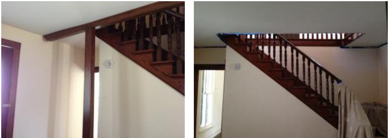
Staircase showing before (left) and after (right). NPS Photo.
