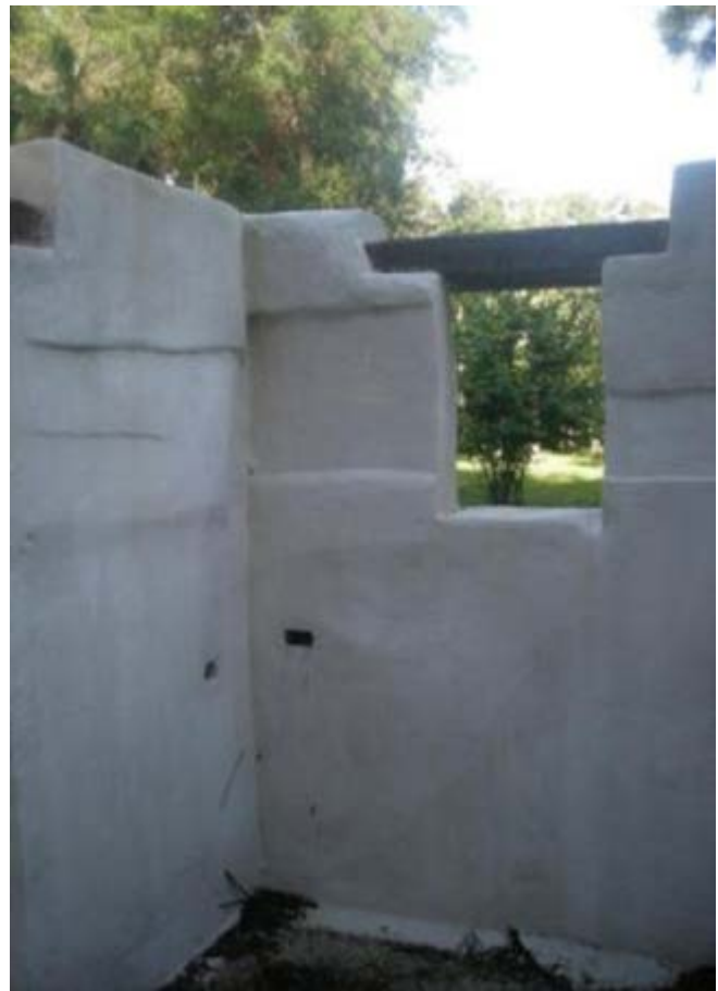
Cabin E14 showing a large crack in the front left wall, top left and bottom left. The picture on the right shows the repair and stabilization of the wall. NPS Photos.
