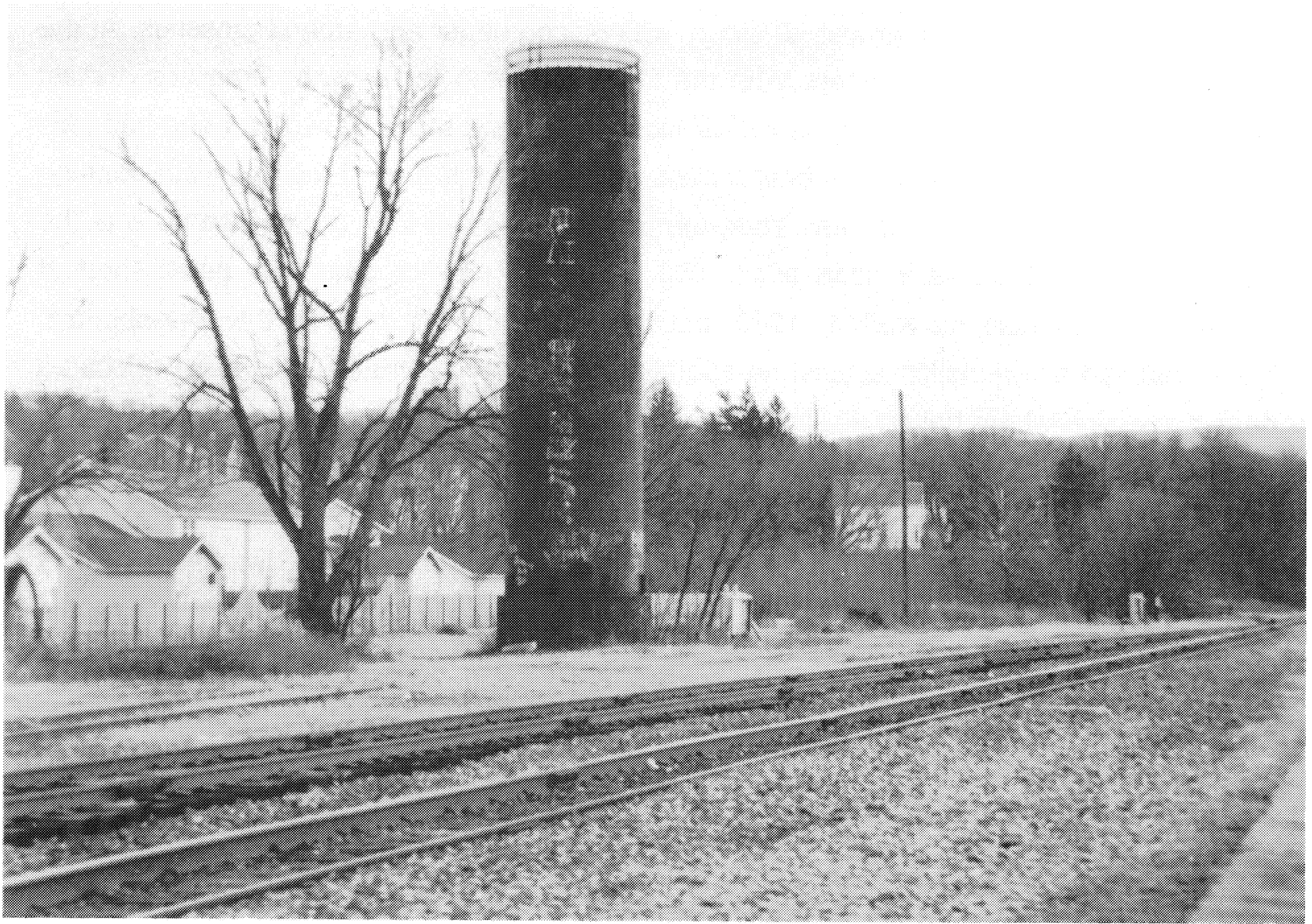
Figure 19 February 1989 East Stroudsburg Water Station
