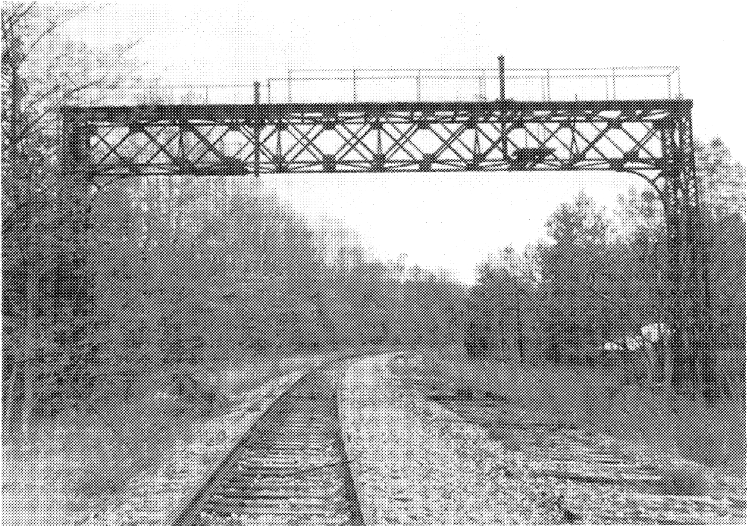
Figure 24 May 1989 Amalomink Signal Bridge
