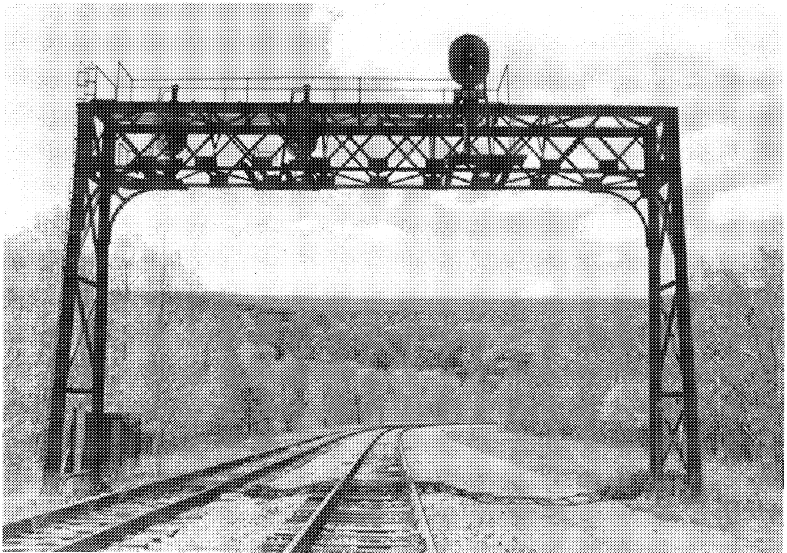
Figure 25 May 1989 Signal Bridge at Mile 125.70
