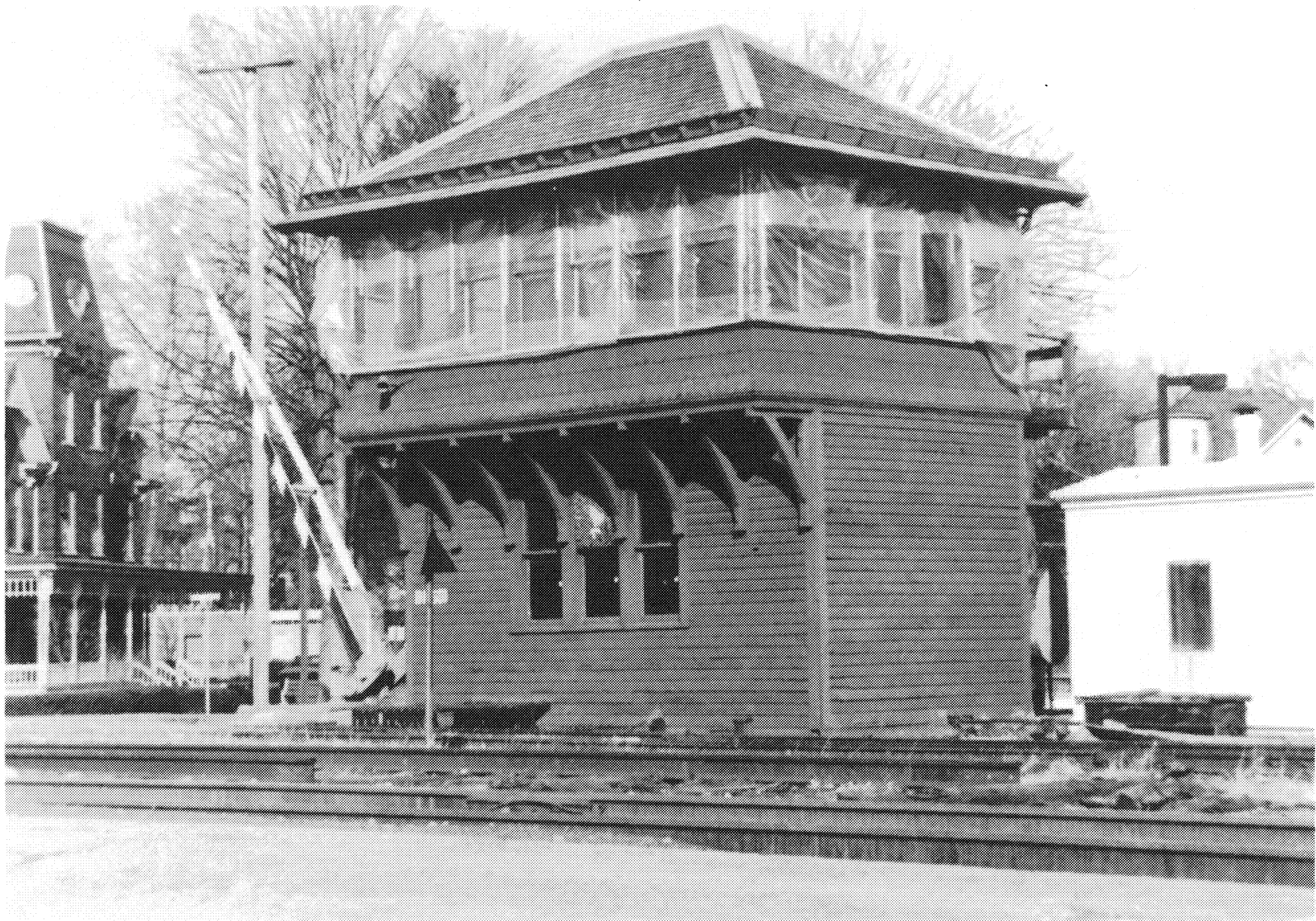
Figure 21 February 1989 East Stroudsburg Interlocking Tower
