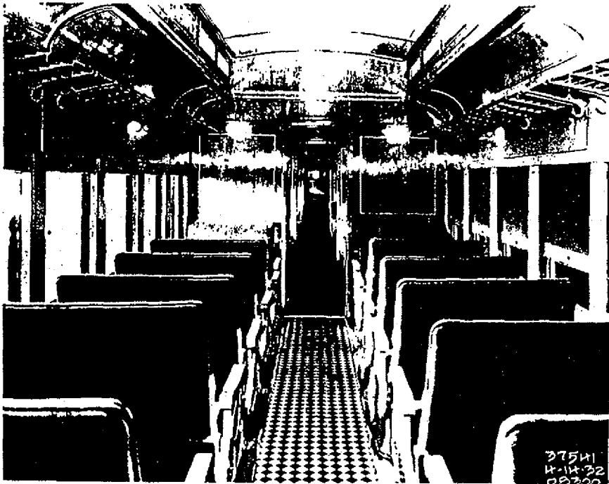
Fig. 3. Interior view of a CNJ passenger coach compartment, showing parcel racks, floor material and walkover seats, 14 April 1932. Photograph No. 30 from the Reading Company Collection, Pictorial Collections and Audiovisual Services Department, Hagley Museum and Library, Wilmington, DE.
