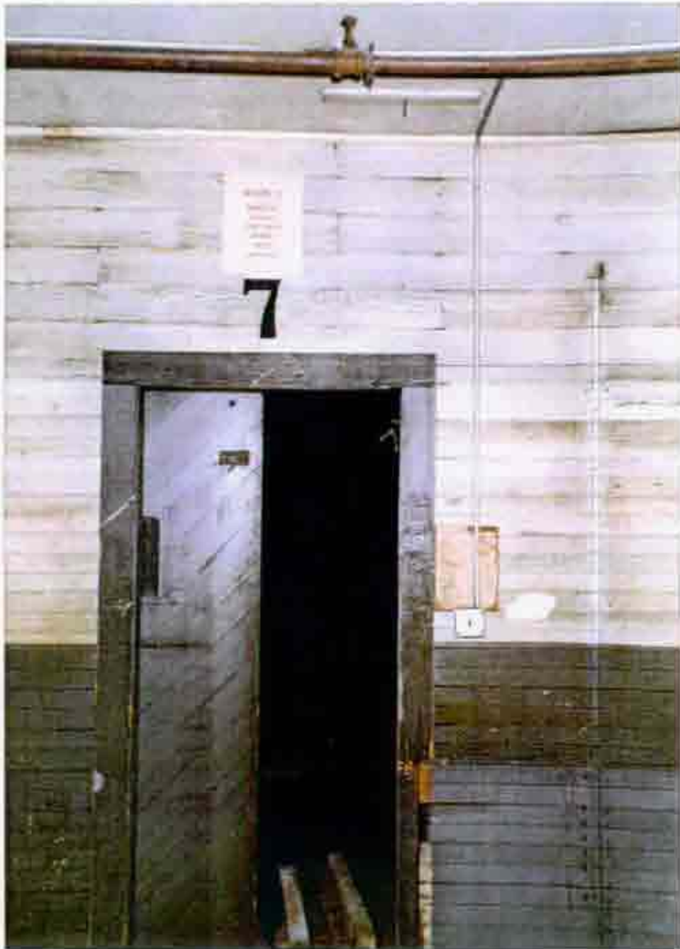
Figure 3.15 Detail of the wood partition and typical door, installed by the Williams Baking Company.
