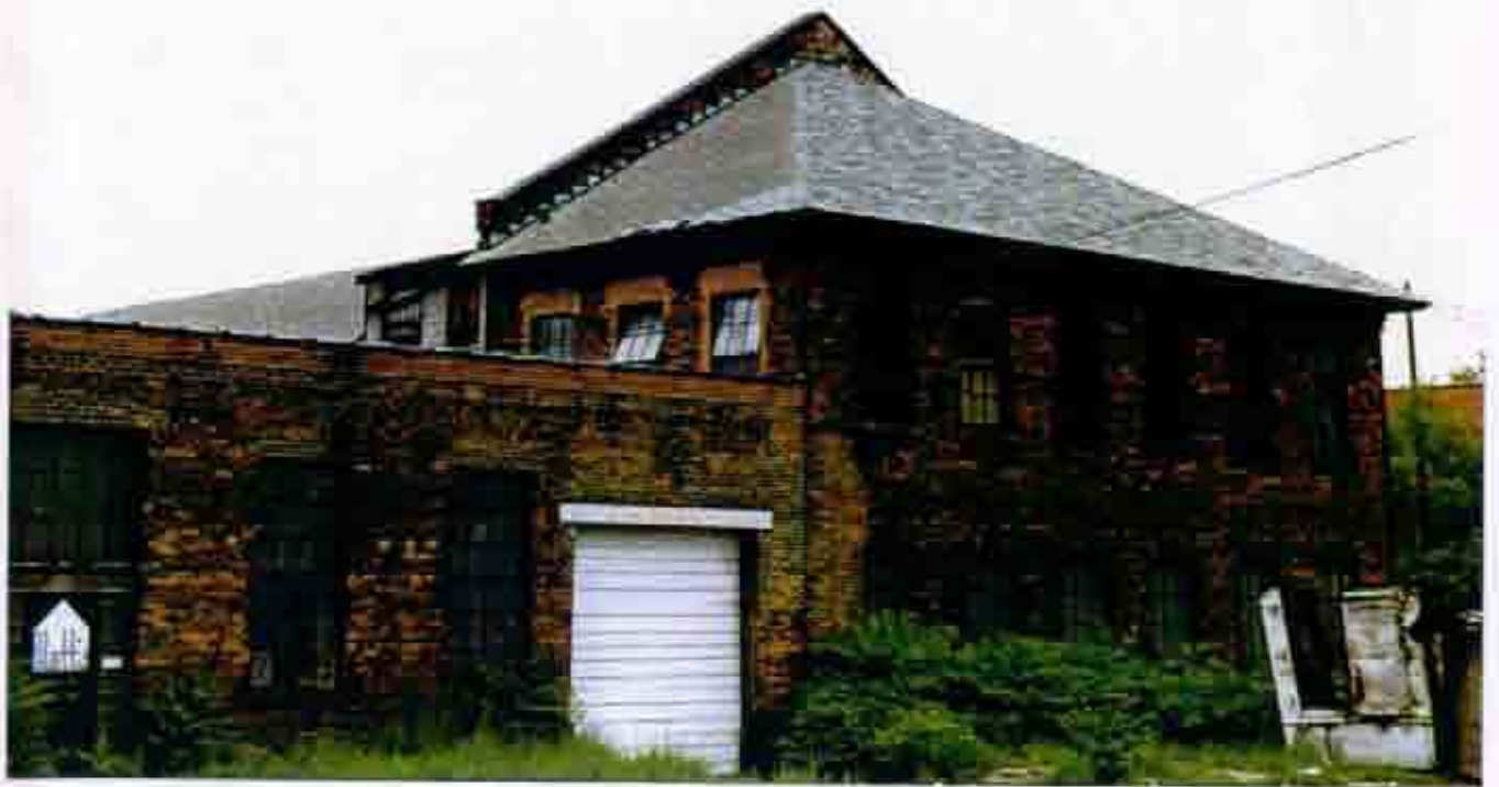
Figure 3.14 Detail of the east elevation of Infill Bay 3 (to the left of Bay 4).
