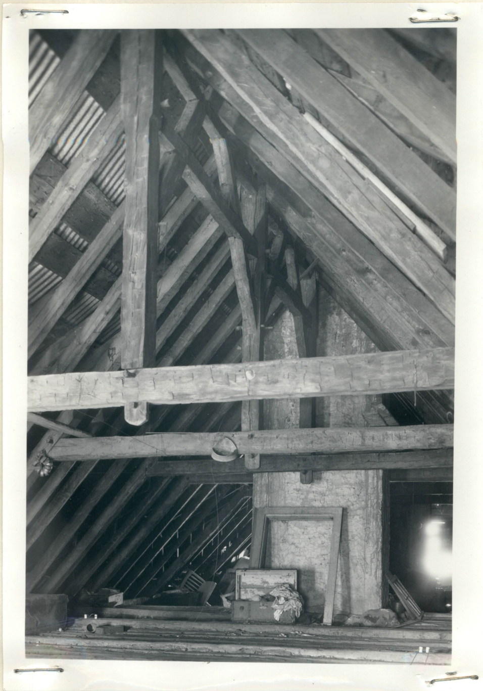
II - C. Bolduc House . Interior of attic, showing Norman trusses and solid log ceiling. Photograph by Charles E. Peterson.
