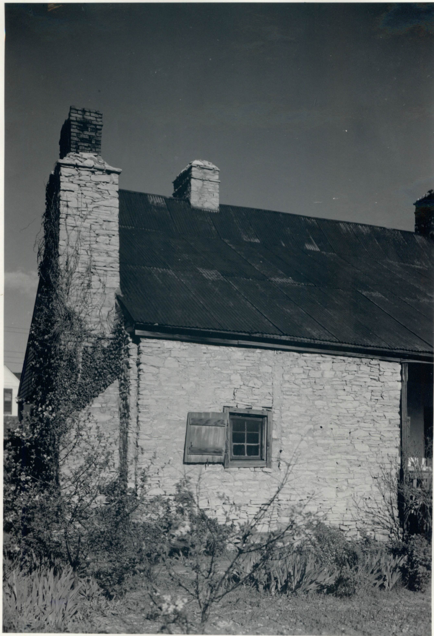
II - B. Bolduc House . Stone kitchen leanto at north end. Photograph by Charles E. Peterson.
