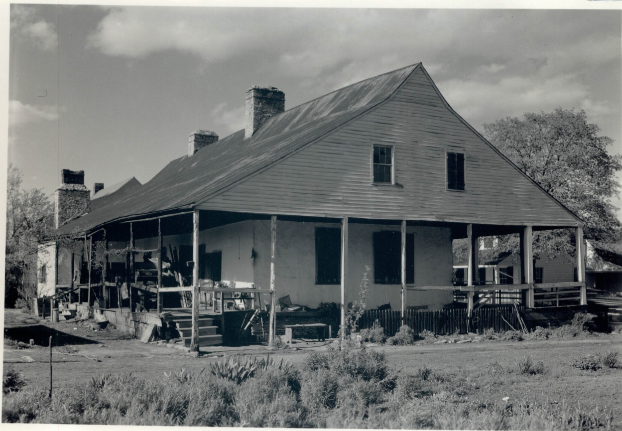
II - A. Bolduc House . General View, showing plastered poteaux sur sole walls and surrounding porch. Structure originally had hipped roof.
