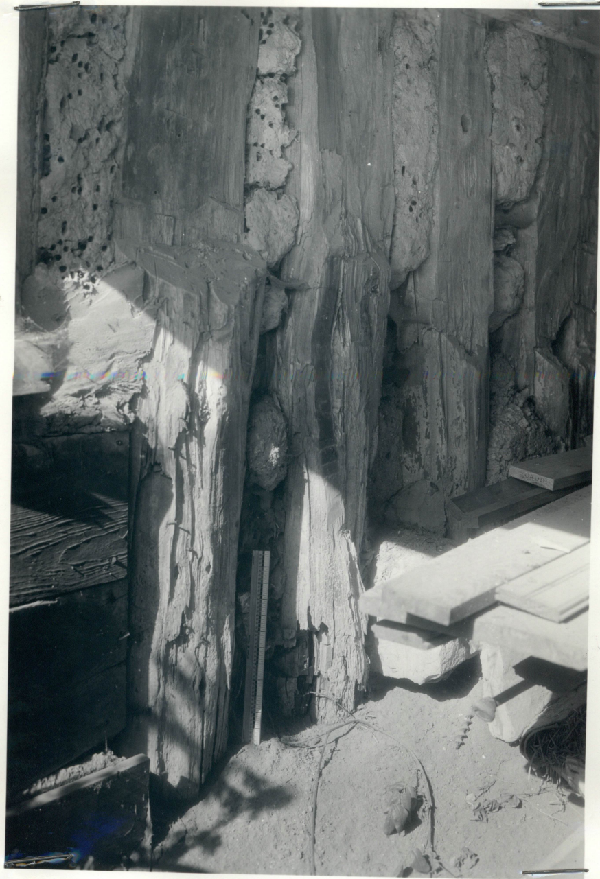
III - B. Ribault House . Detail of palisadoed or poteaux en terre construction. Cedar logs bougillé with clay and grass. Photograph by Charles E. Peterson.
