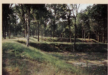
Curtain Wall No. 2 and traverse, Fortress Rosecrans
