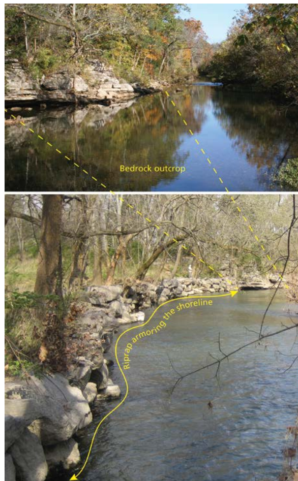
Figure 11. Riprap installed adjacent to bedrock outcrops along the West Fork Stones River. Visitors frequently recreate in this area, using the riprap surfaces as fishing perches. Note the location of bedrock outcrops in the magnified view along the river edge. Photograph by Trista L. Thornberry-Ehrlich (Colorado State University) in March 2009.
