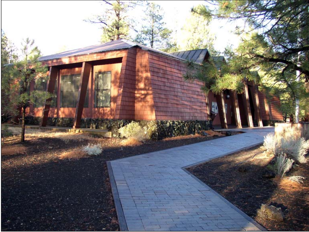
Figure 6. Sunset Crater visitor center, looking west (NPS 2003). Note windows and walkway.
