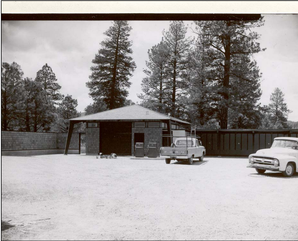
Figure 7. Maintenance area before carport was enclosed (NPS 1967).
