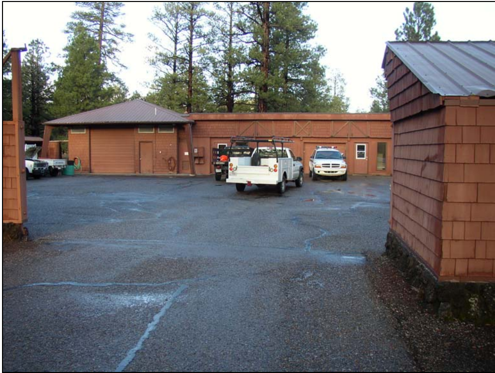
Figure 8. Maintenance area after carport was enclosed (NPS 2003). Also note shed in right foreground, also added in the early 1980s.
