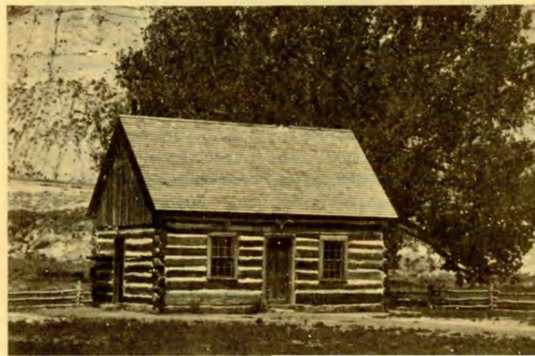
Restored Maltese Cross cabin.
