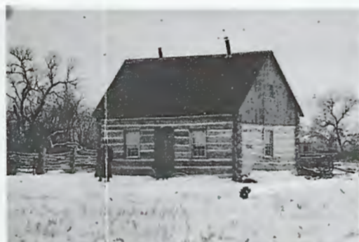
The Maltese Cross cabin, the main house on Roosevelt's ranch, was a substantial, soundly built structure.
