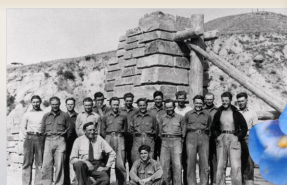
We still benefit today from the work of the Civilian Conservation Corps. These young men built the park's roads, culverts, trails, and structures in the 1930s. Right: Blue penstemon, prairie wild rose, sunflower, and crested beardtongue.
