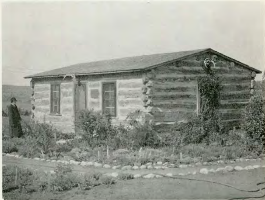
The Maltese Cross cabin on the State Capitol Grounds.
