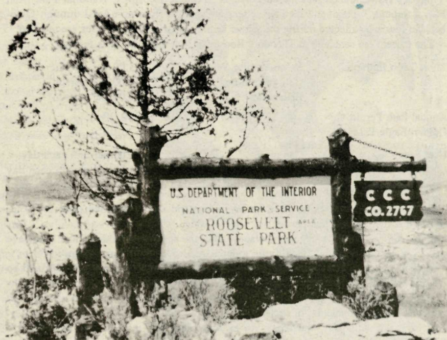
The 1930s CCC camps were located in what would later become the South and North Units of the Park.
