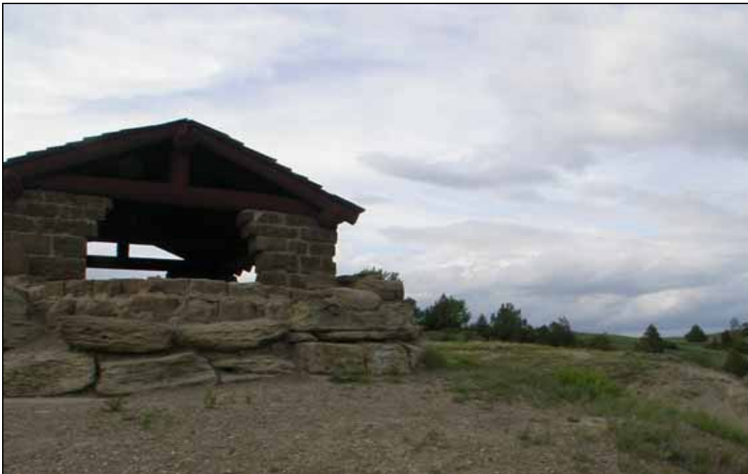
Figure 15. Shelter at Riverbend Overlook. The Civilian Conservation Corps used medium-grained, cross-bedded sandstone from a local quarry to construct various structures in the park, such as this shelter in the North Unit. NPS photo by Dave Krueger.
