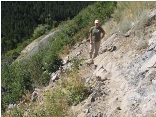
Before: Pine Hollow Trail tread has eroded away along the cliff face.
