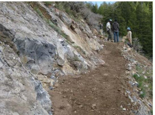
After: Blasting along the cliff face creates a safe tread width along Pine Hollow Trail.
