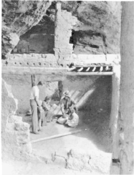
Notice part of original roof over the room on right side
