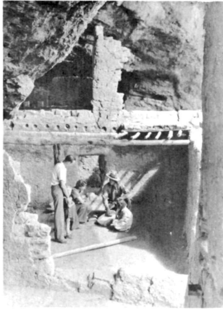
Notice part of original roof over the room on right side
