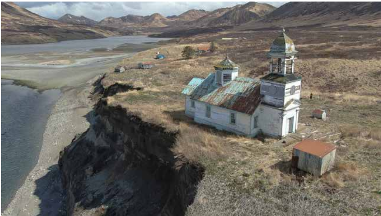
[13] The Church of Our Lord Chapel, Karluk, AK, was built in 1888 and is the oldest Russian Orthodox Church in Alaska. In danger of collapse into the Karluk River, the erosion of the bluff has been rapidly escalating, and the church sits only 25 feet from the edge. The vulnerability of the property at the edge of a river requires frequent monitoring, but a more long-term solution will be necessary for the continued preservation of the building. Photo: Tom Pillifant
