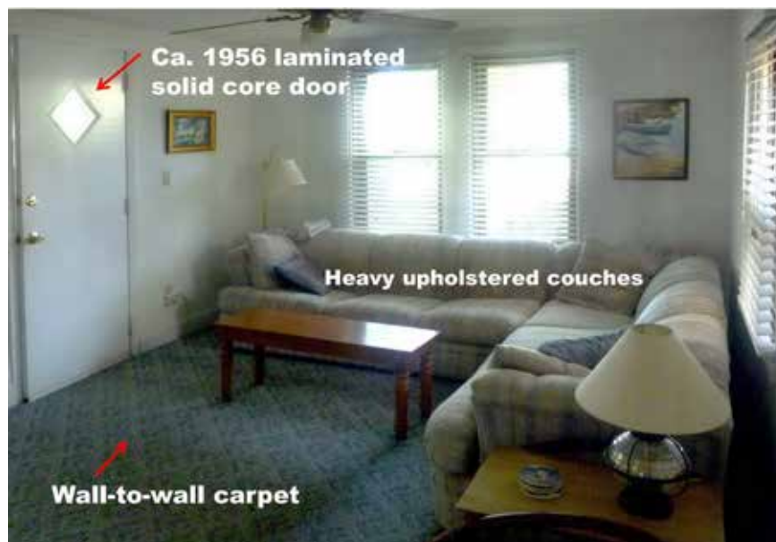
Figure 6: The living room before Hurricane Sandy included non-historic wall and floor finishes. Windows and doors were also non-historic and made of materials that absorbed floodwater, warped, and/or could not easily be cleaned. Photo: Mary Delaney Krugman, JD, MSHP
