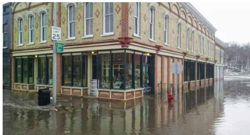
Figure 7: Floodproofing measures kept the water out of the Driver Opera House during a 2019 flood. Photo: Brian Mesmer
