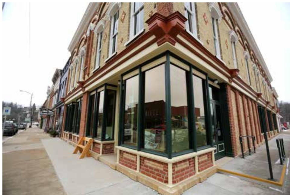
Figure 6: Exterior of the building after the dry floodproofing project is complete. The exterior steel storefront framing is a historic feature, painted green above the storefront and cream below after rehabilitation. Photo: Dave Kettering/Telegraph Herald
