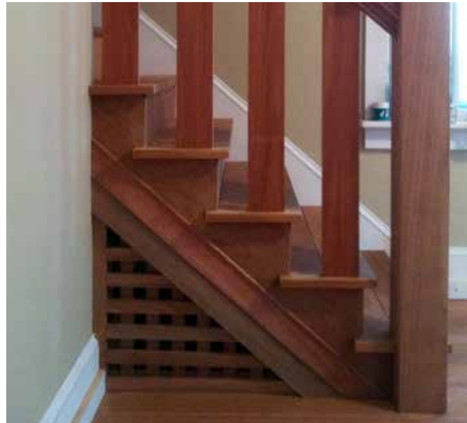
Figure 3: Instead of solid wall material, an open lattice was installed under the stair to vent an otherwise inaccessible space. Photo: Mary Delaney Krugman, JD, MSHP
