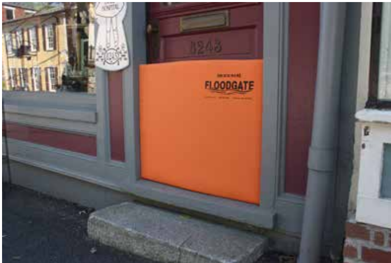
[22] This floodgate is a temporary solution that can only be deployed with enough notice of a potential flood event. Storage of the gate apparatus must be on or close to the property with ready access in order to be actively deployed. Photo: Liz Petrella/NPS
