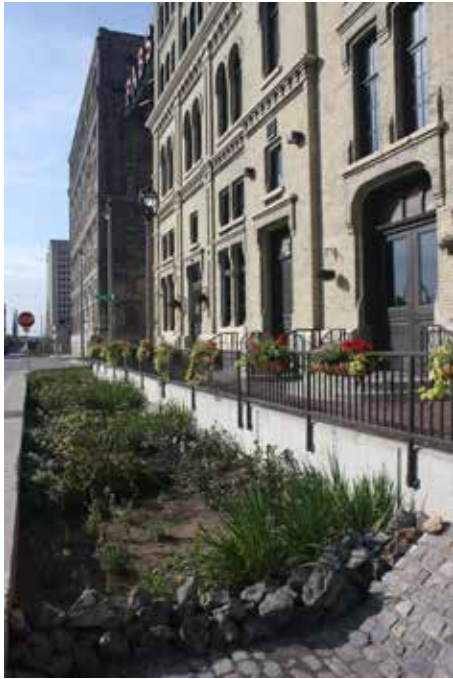
[39] Street and sidewalk improvements that include bio-swales or other water retention systems can be effective devices to collect or direct water and alleviate flooding as shown here in Milwaukee, WI. Photo: Liz Petrella/NPS
