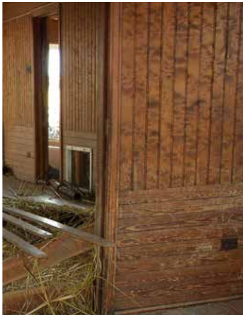
[17] (a) Interior woodwork at the Charnley-Norwood House, known as Bon Silene, in Ocean Springs, MS, withstood a storm surge of 30 feet from Hurricane Katrina in 2005. Interior walls, ceilings, and cabinetry are constructed of curly heart pine. Milled from the heart of Longleaf pine trees, heart wood is known to be insect and rot resistant. (b) The restoration project, which included repairs to the interior wood paneling, was completed in 2014.
