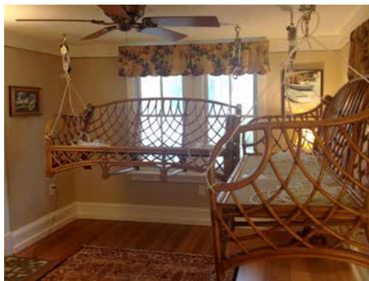
Figure 8: A pulley system lifts heavy or bulky furniture above predicted flood waters. All other contents can be moved to upper levels of the house. Photo: Mary Delaney Krugman, JD, MSHP
