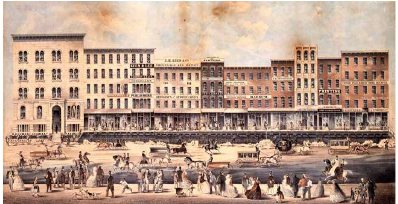
[74] Elevating masonry buildings built to the side lot lines can be difficult but has been done historically. This illustration shows an entire merchant block in Chicago being elevated at one time in 1857, as part of a larger plan to elevate the entire downtown area by four feet. Photo: Chicago History Museum, ICHI-059709
