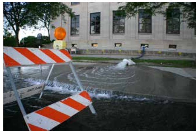
[65] Flood waters often must be actively pumped out of and away from the property, as seen in this image from Des Moines, IA. The pumping process should be designed to control the shift in hydrostatic pressure on the building and remove all flood waters that do not naturally drain or recede from the property. Photo: Chris Snider
