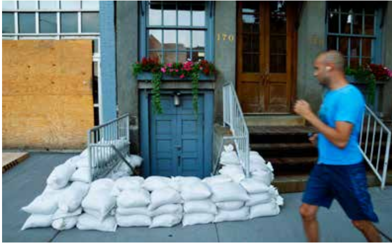
[20] Temporary measures such as sandbags can be a simple and inexpensive solution for protecting buildings in low-lying and vulnerable areas, but they are not meant to withstand moving floodwaters for extended time periods. Photo: Eduardo Munoz/Reuters
