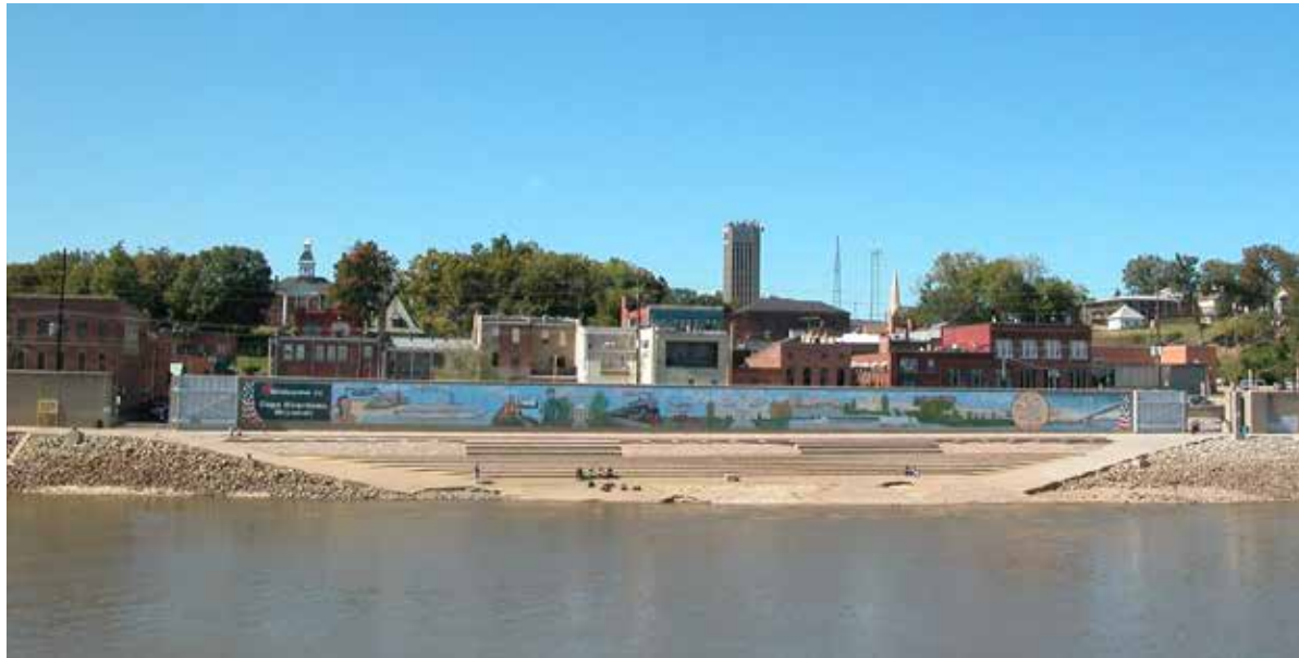
[33] A large floodwall protects the historic downtown of Cape Girardeau, MO, from the Mississippi River. Photo: VisitCape
