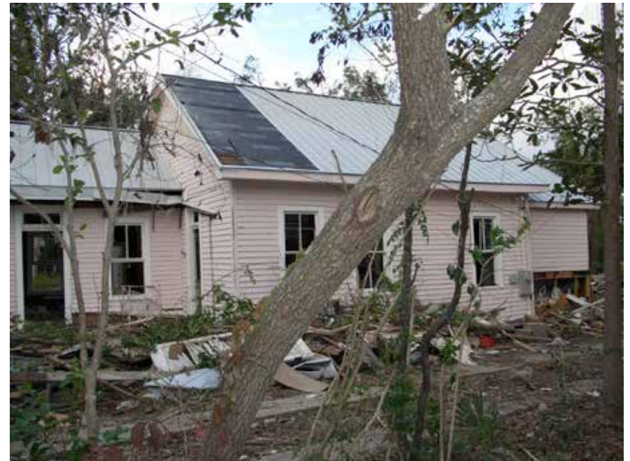
Figure 4: This photo of the hurricane damage shows that part of the roof was stripped away, and debris littered the site around the house. Photo: Mississippi Department of Archives and History, Mississippi Historic Resources Inventory (HRI) Database. http://www.apps.mdah.ms.gov/Public
