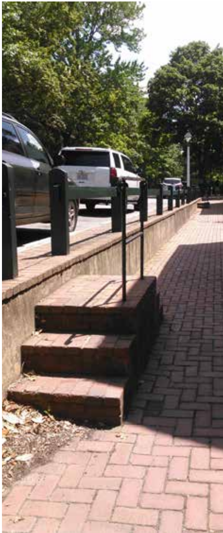
[36] Raised streets may require additional access points to residential and commercial properties if the sidewalks and buildings are not also raised. This 1890s historic example from Old Salem, NC, incorporated new brick stairs and railings. Additional considerations for accessibility would need to be addressed today. Photo: Jennifer Wellock/NPS
