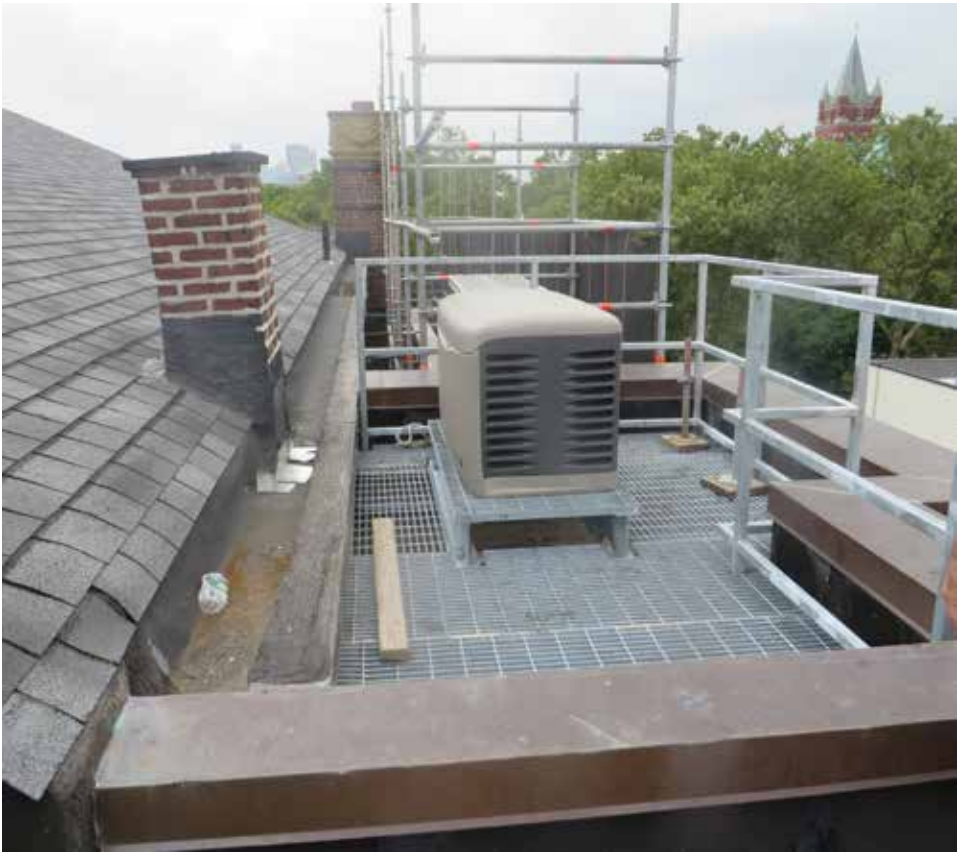
[46] For many buildings in flood-prone areas, having a generator on site may be a necessity to provide emergency power for pumps and other mechanical equipment. This public library in Hoboken, NJ, has a generator located on a flat roof high above any flood waters and not visible from the street. Photo: David V. Abramson for Hoboken Public Library
