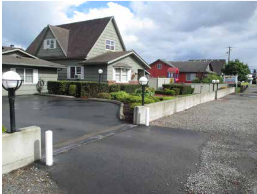
[30] This low-scale floodwall in Washington state provides flood protection without compromising the historic character of the property or obstructing views of the historic house from the street. A deployed floodgate can seal the opening at the driveway during a flood event. Photo: French Wetmore
