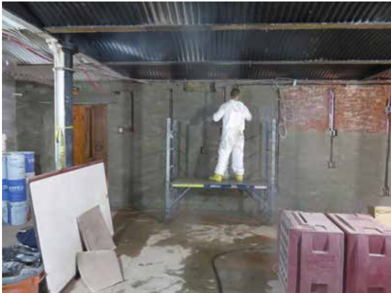
[48] A waterproof coating is applied to the interior surface of lower-level walls of the public library in Hoboken, NJ. Prior to applying such a coating, the product should be researched by building science professionals with knowledge of historic materials and methods to ensure that the coating will not cause damage to or accelerate deterioration of the structure. Photo: David V. Abramson for Hoboken Public Library
