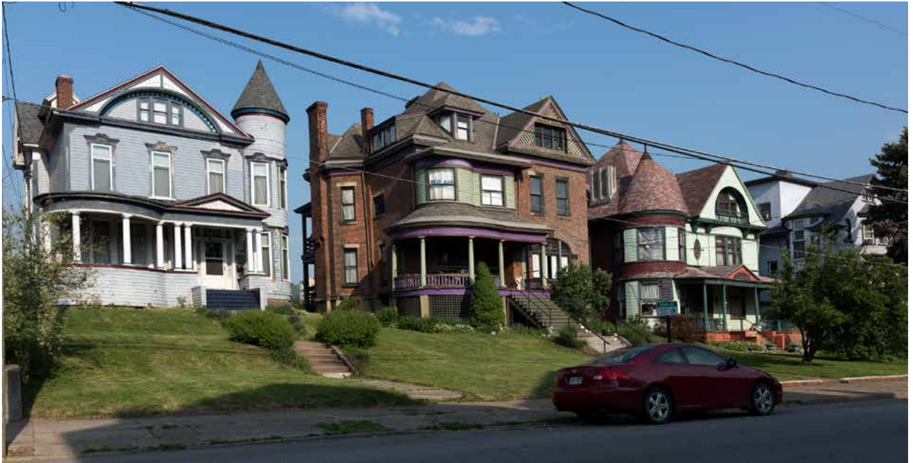
[78] In many areas that have a history of flooding, buildings may have already been raised. Wheeling Island in the middle of the Ohio River in Wheeling, WV, was inundated by thirty-three floods between the 1860s and 1960s. During this period buildings on the island were constructed on tall foundations or were lifted onto higher foundations or berms after flood events. Photo: Library of Congress, Prints & Photographs Division, photograph by Carol M. Highsmith (altered)
