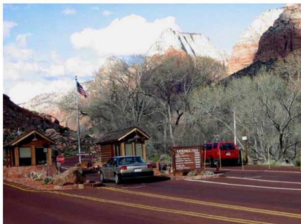
Zion Entrance Station – Red SUV in Automated Lane (right hand lane)
