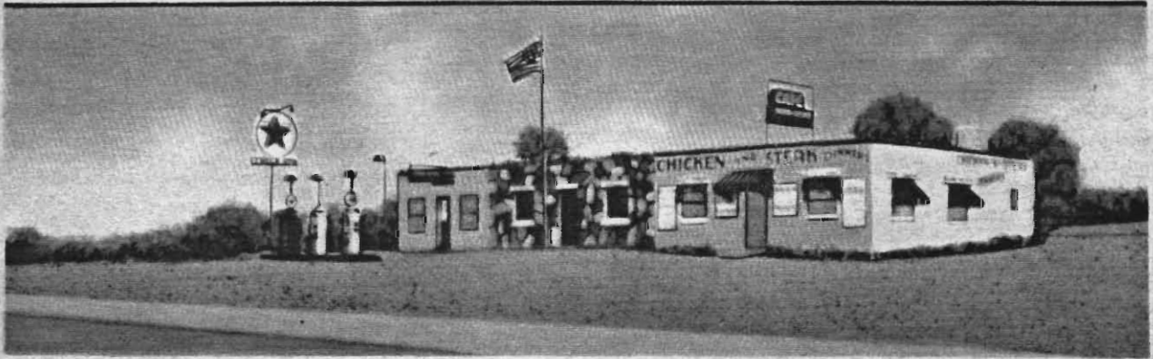
1 MILE EAST OF LEBANON, MO., ON HIGHWAY 66.
