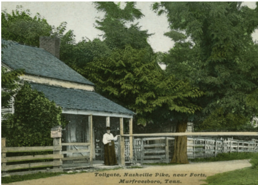
Tollgates, such as the one shown here, were located at various points on turnpikes in order to collect tolls. Courtesy of MTSU Center for Historic Preservation.
