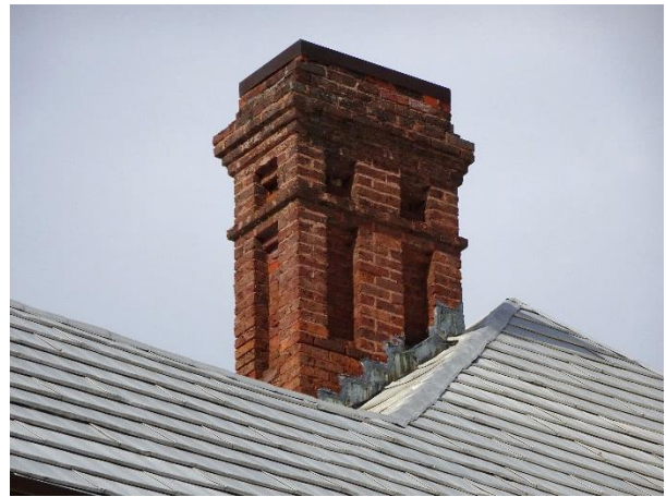
FIGURE 18. Typical brick chimney with corbelled brick details.
