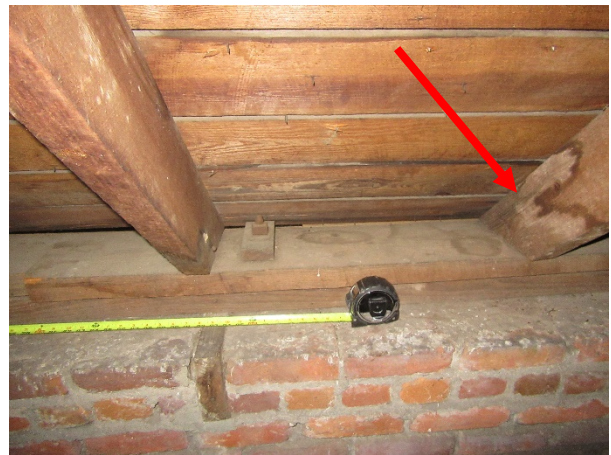
FIGURE 71. Moisture staining at roof rafters.
