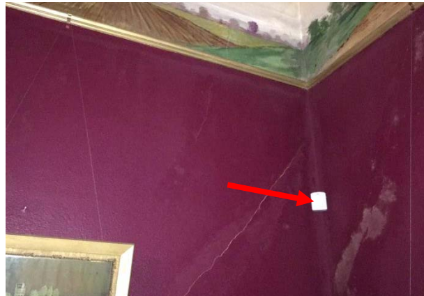
FIGURE 185. Typical security motion sensor.
