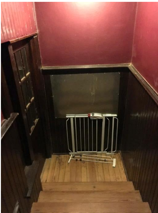
FIGURE 151. Sheet-metal closure at rear hall stair.
