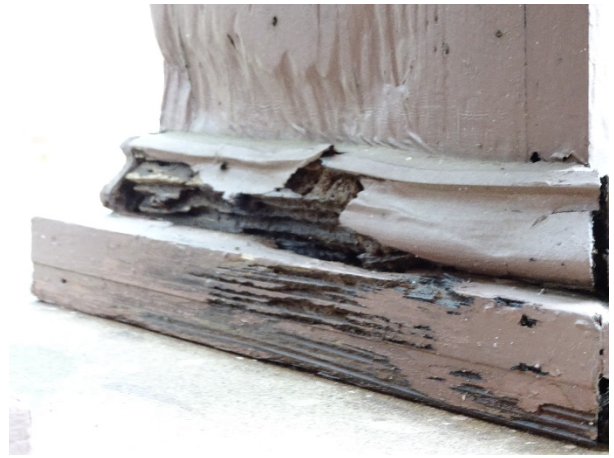
FIGURE 43. Deteriorated wood at base of columns.
