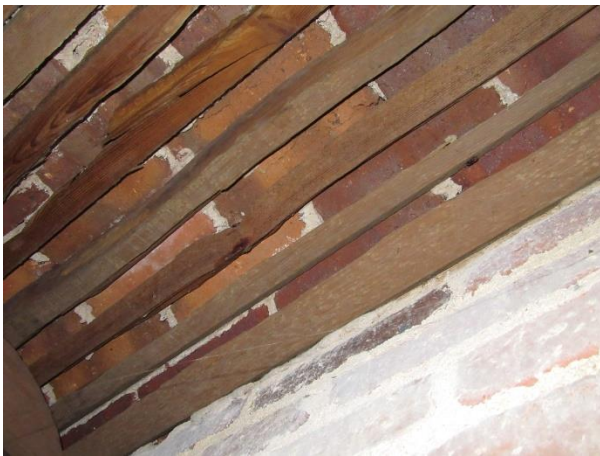
FIGURE 133. Typical masonry infill with wood slats shoring at underside of hearth.
