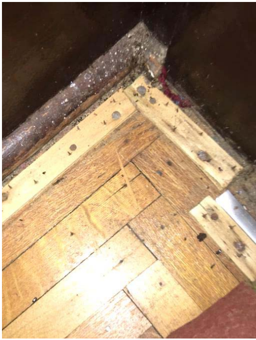
FIGURE 120. Original wood flooring below carpet at vestibule.
