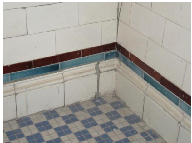
FIGURE 102. Detail at tile wall base.
