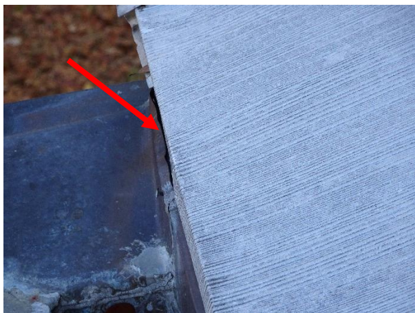
FIGURE 66. Gap between the copper flashing and the roof cladding.
