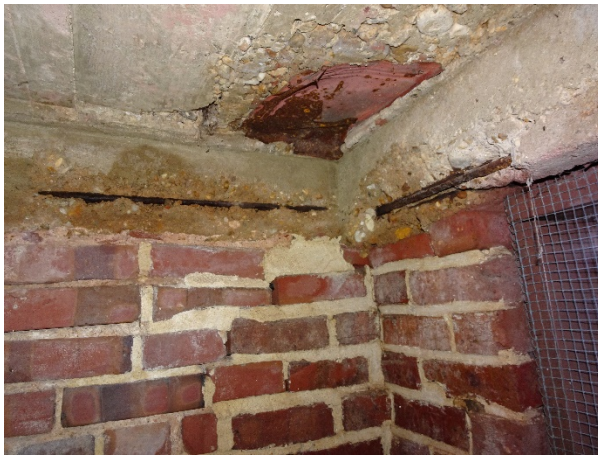
FIGURE 30. Spalled concrete bond beam at porch wall.
