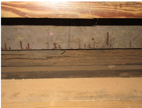
FIGURE 165. Termite damage at basement framing.
