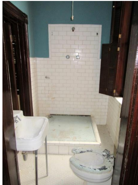
FIGURE 178. Overall view of Portia's shower.
