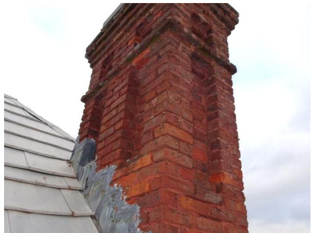
FIGURE 21. Deteriorated mortar joints and evidence of previous repointing efforts visible at the chimney.
