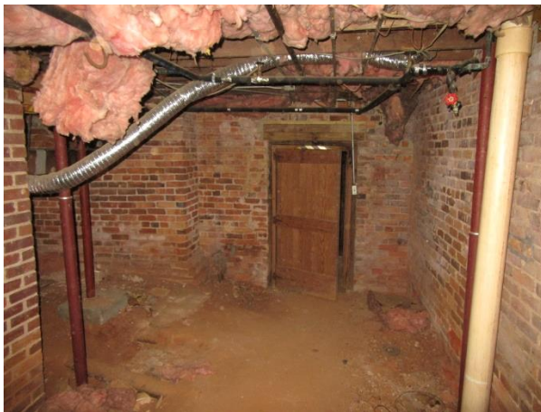
FIGURE 164. Overall view of mechanical crawl space / basement.
