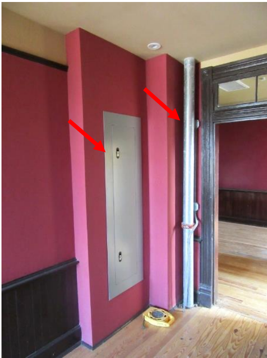
FIGURE 182. Electrical panel and sprinkler standpipe at west bedroom.
