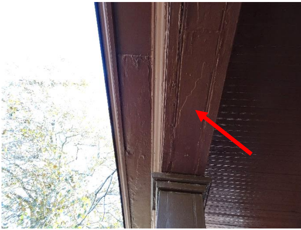
FIGURE 46. Previous paint coatings at wood porch members were not completely removed prior to repainting.
