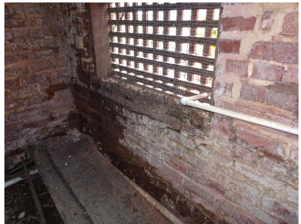
FIGURE 28. Evidence of moisture infiltration at northwest corner of porch.
