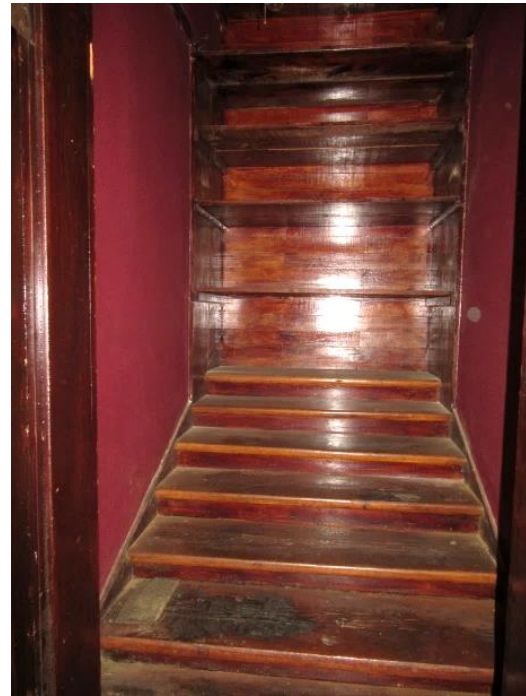
FIGURE 140. Shelving infill at second floor stair.
