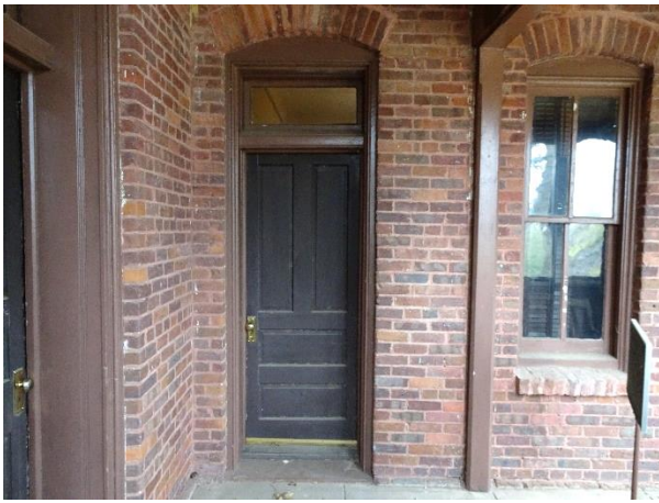
FIGURE 51. Typical side door with four solid panels.
