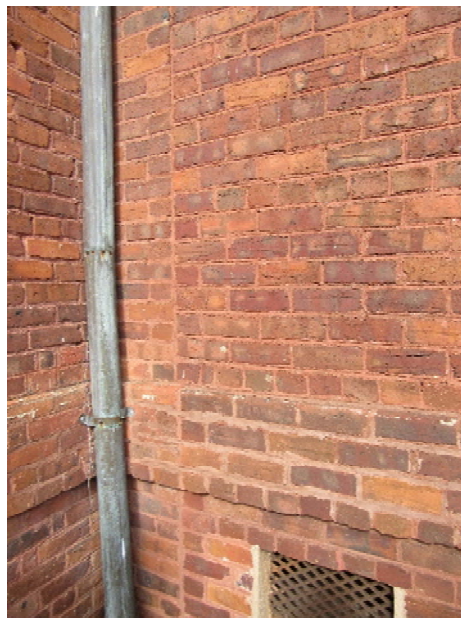
FIGURE 16. The corner where the dining room addition abuts the main structure.
