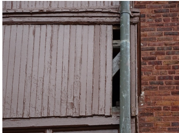
FIGURE 39. Missing wood cladding at south two-story porch.
