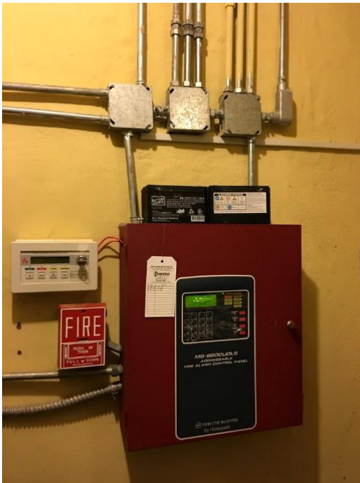
FIGURE 183. Fire-alarm control panel at guest room closet.
