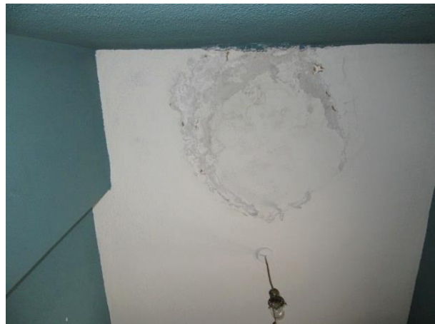
FIGURE 99. Second-floor shower (Room 203) - plaster damage at ceiling.
