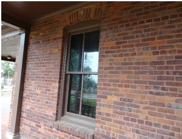
FIGURE 49. Typical masonry window.
