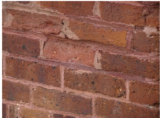
FIGURE 22. Evidence of previous mortar repointing in the field of wall.
