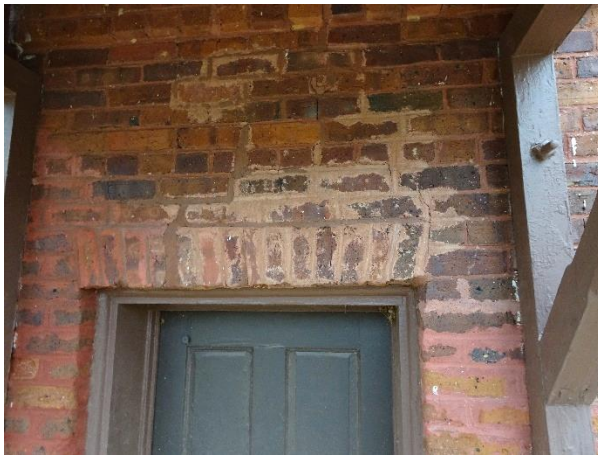
FIGURE 54. Cracking and open mortar joints above flat arch opening.
