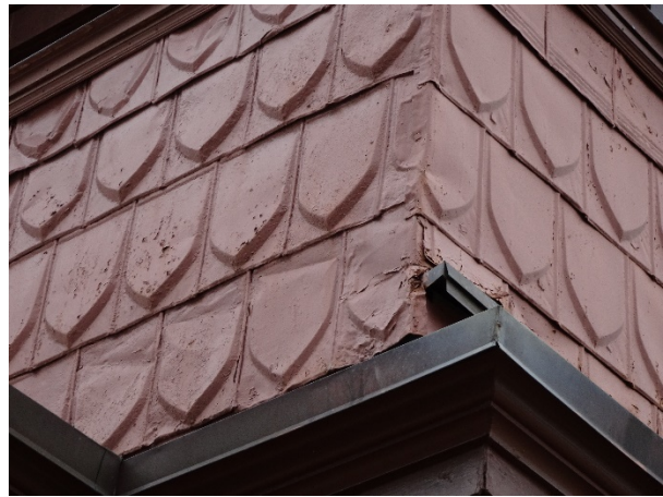
FIGURE 35. Peeling paint at pressed sheet-metal cladding.
