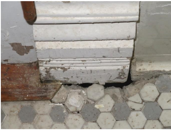
FIGURE 131. Tile damage at door frame.
