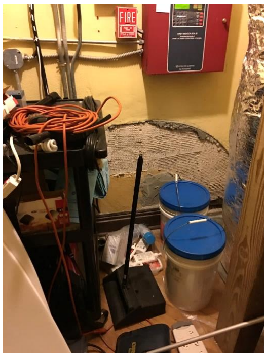
FIGURE 104. Plaster damage in the guest room closet.
