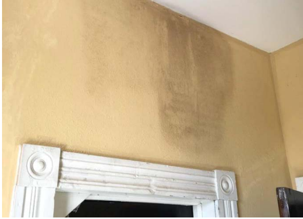
FIGURE 100. Mold / mildew stain at third-floor wall surfaces.
