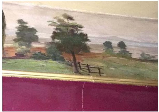
FIGURE 115. Previously repaired crack at mural where retouched paint is not visible.
