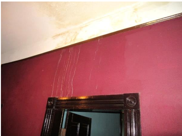
FIGURE 95. Plaster damage from water at second-floor front hall.
