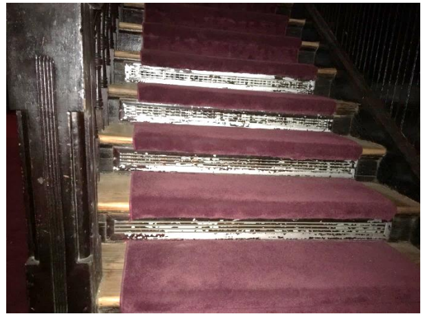
FIGURE 175. Return air grilles on stair risers.
