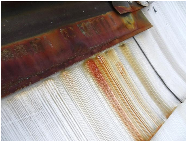
FIGURE 75. Corrosion staining at interface of flashing with roof cladding.
