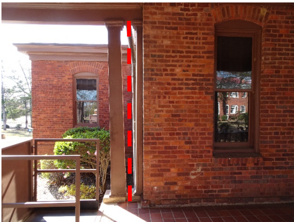
FIGURE 48. Tilted and displaced porch column.
