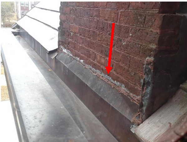
FIGURE 74. Deteriorated sealant at regletted flashing joint.
