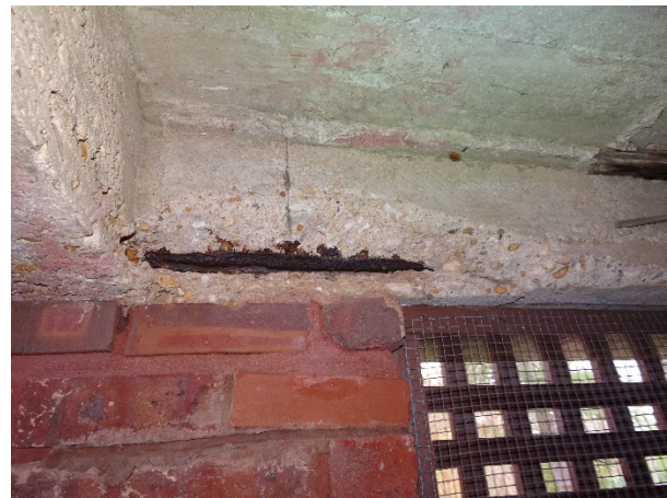
FIGURE 29. Spalled concrete bond beam at porch wall.
