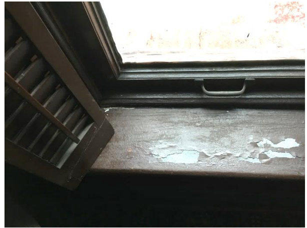
FIGURE 148. Paint delamination at window stool.
