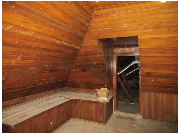
FIGURE 138. Typical stained wood interior at third-floor trunk storage rooms.
