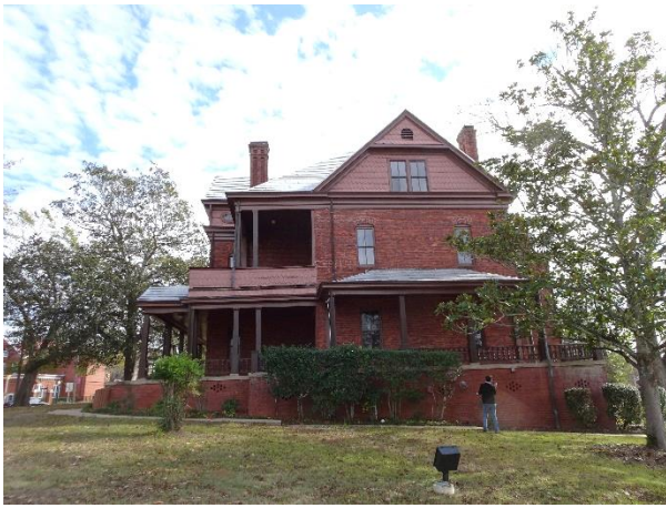
FIGURE 5. The Oaks, west elevation, looking east.
