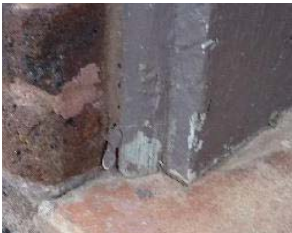
FIGURE 56. Peeling paint at door and window framing members.
