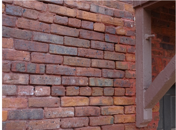
FIGURE 15. Typical brick exterior wall.
