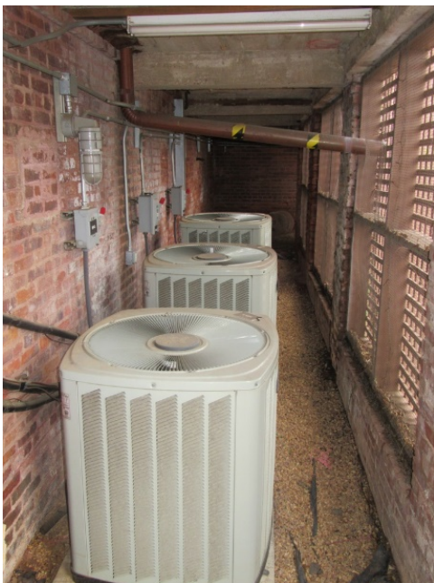
FIGURE 169. Condensing units at porch crawl space.
