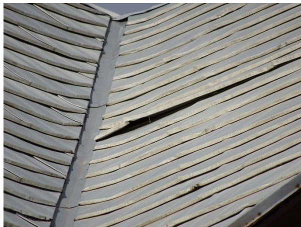
FIGURE 69. Bowed and displaced sheet metal at field of roof.
