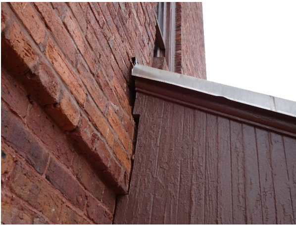
FIGURE 40. Displaced roof framing over south entrance.
