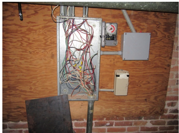
FIGURE 199. Open make-up box in basement.
