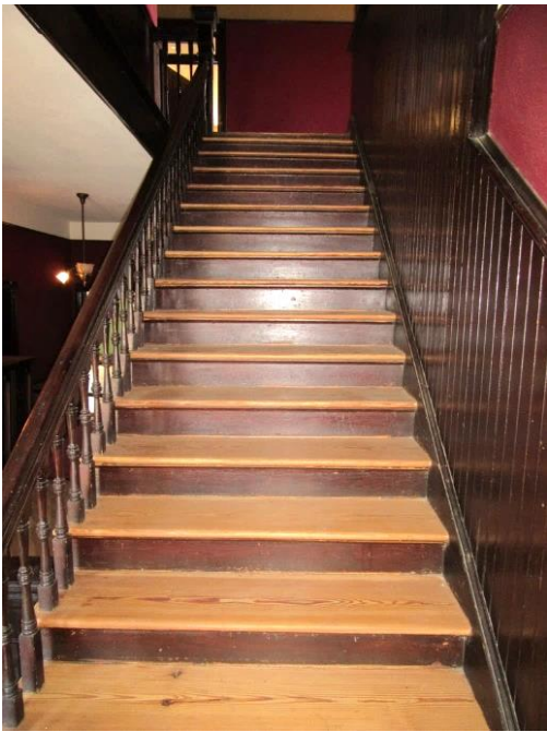
FIGURE 124. Stair from second to third floor.
