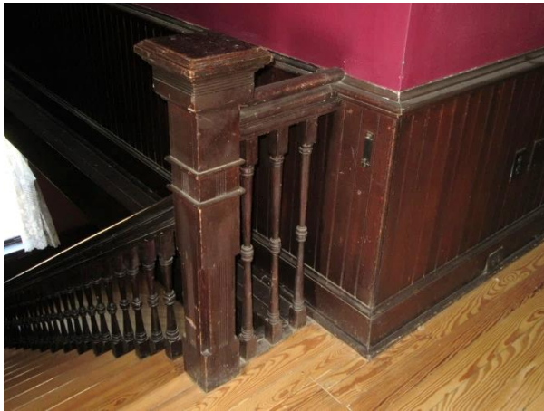
FIGURE 146. Common damage to balustrade rail and newel post on the third floor.
