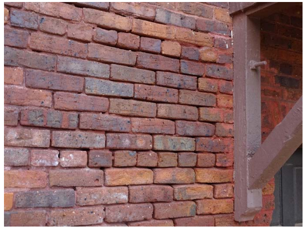
FIGURE 20. Eroded mortar joints at the field of the wall.
