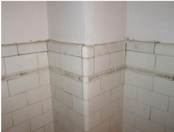
FIGURE 101. Detail of wall tile at bathroom.
