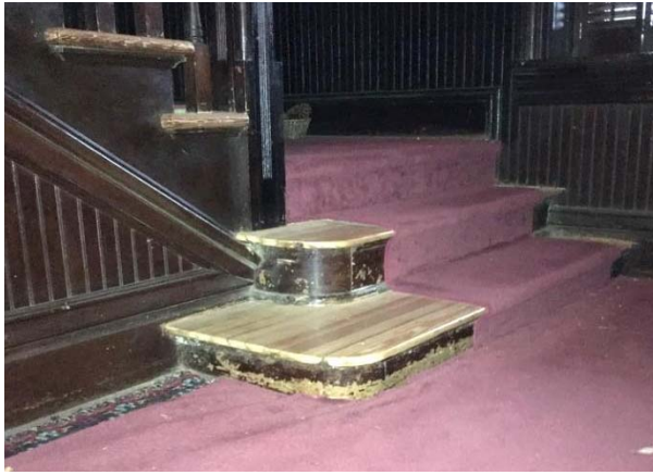
FIGURE 144. Paint deterioration at stair risers.
