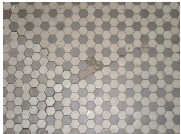
FIGURE 129. Cracks in mosaic floor tile at bathroom.
