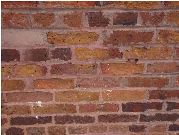
FIGURE 25. Face spalling of brick.
