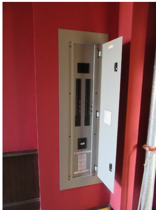
FIGURE 198. Electrical sub-panel in west bedroom.
