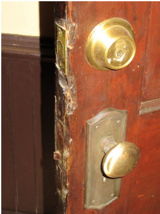
FIGURE 159. Detail of hardware on the third floor.
