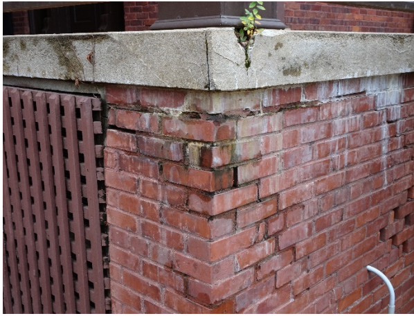
FIGURE 23. Step cracking, open joints, and evidence of water infiltration at the porch walls.
