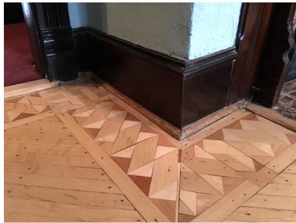
FIGURE 119. Parquet border at second floor.
