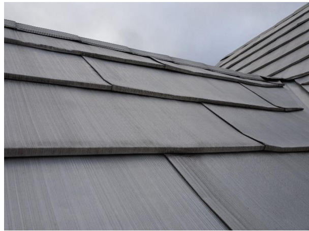
FIGURE 59. Detail of pressed sheet-metal roofing with grooved pattern, giving the appearance of a wood shingle.
