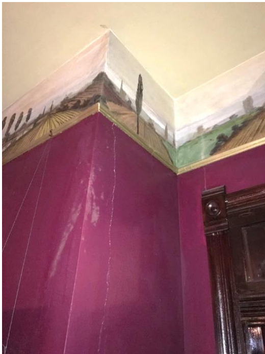
FIGURE 91. Paint damage at dining room.
