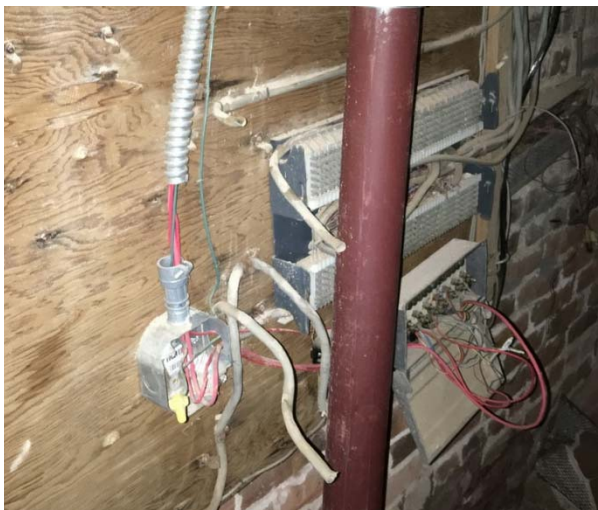
FIGURE 201. Open junction box and panel at telephone backboard, basement.
