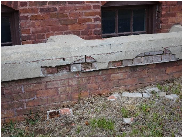
FIGURE 19. Spalling of the brick and cementitious parge coating at the light well walls.
