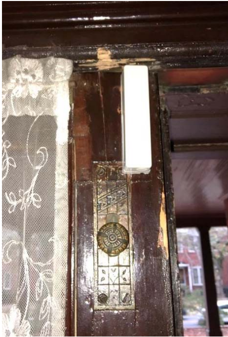
FIGURE 152. Flushbolt at head of inactive leaf at entry. Stile is split from heavy use.
