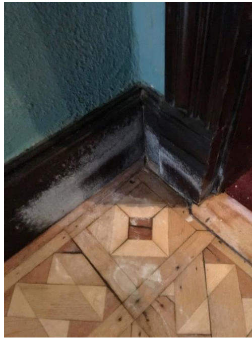
FIGURE 125. Moisture damage at floor and base.
