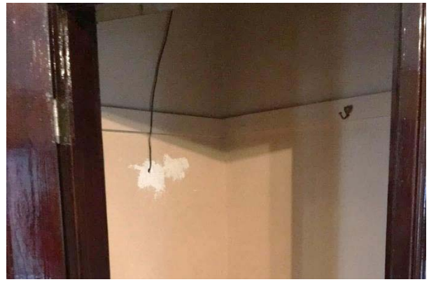
FIGURE 188. Wall penetration at low voltage wiring in closet.
