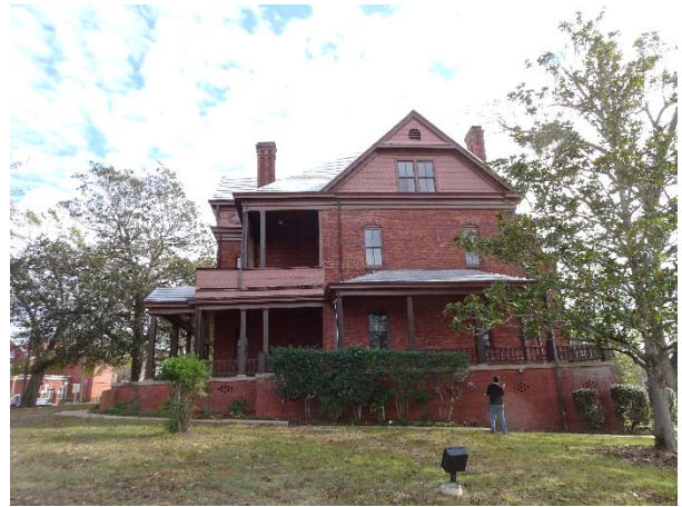
FIGURE 37. The Oaks, west elevation, looking east. Note the second-floor balcony at the left.
