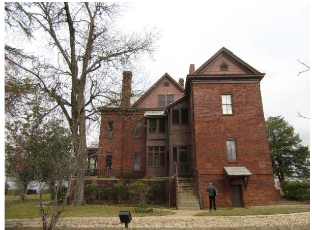
FIGURE 38. The Oaks, south elevation, looking north showing the two-story, screened-in porch.
