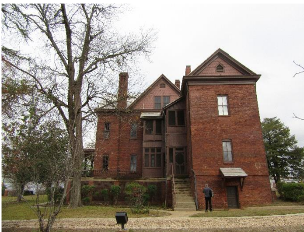
FIGURE 7. The Oaks, south elevation, looking north.
