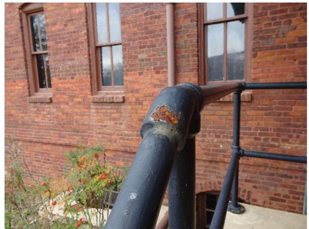
FIGURE 58. Surface corrosion and paint loss at metal handrail.
