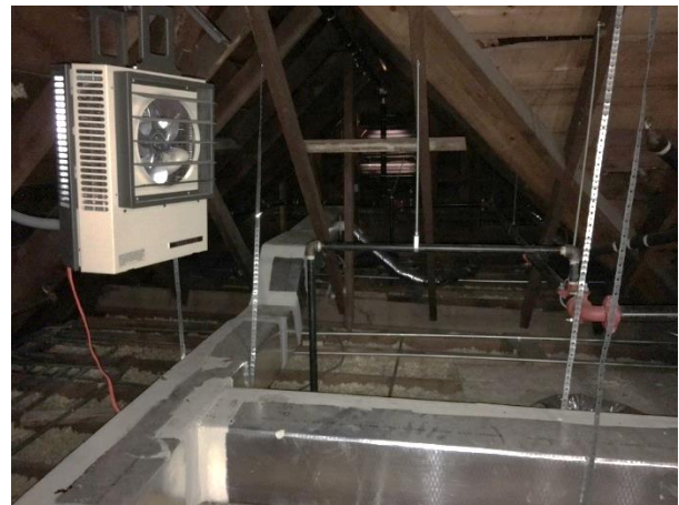
FIGURE 171. Electric heater at attic.
