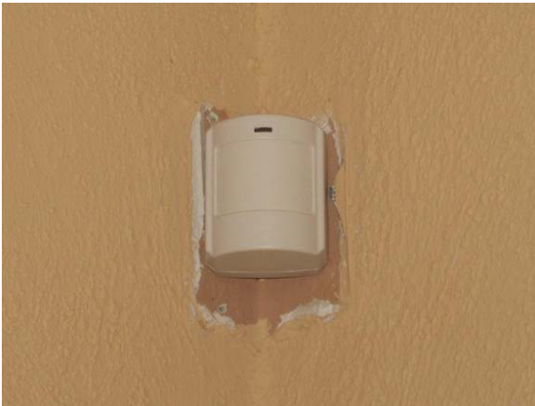
FIGURE 187. Paint incomplete where device has been replaced.
