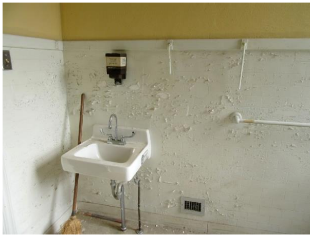
FIGURE 103. Lavatory and painted wainscot in the third-floor bathroom.
