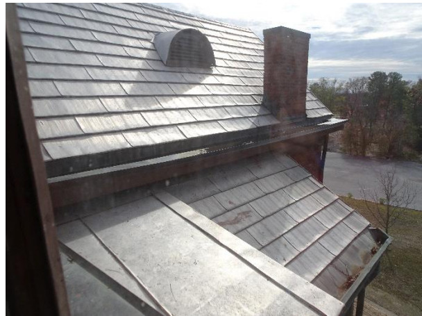
FIGURE 60. Typical roofing material, plus the standing seam panel and aluminum roof vent.
