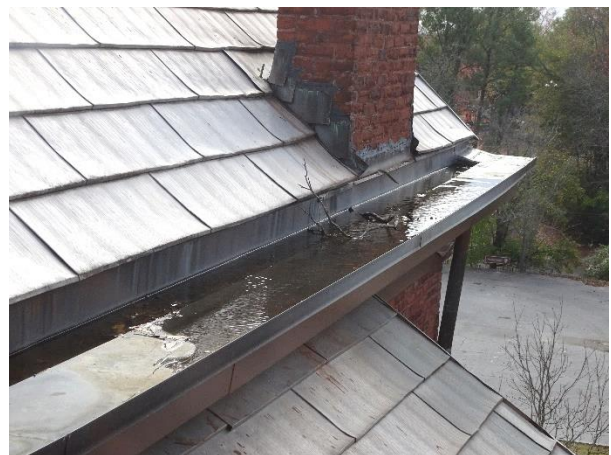
FIGURE 63. Gutter overflowing with water. Note branches in the gutter.
