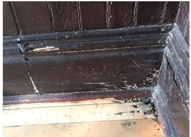
FIGURE 149. Deterioration due to moisture damage in the kitchen.
