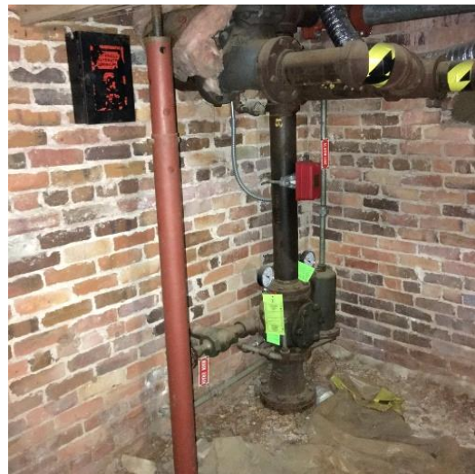
FIGURE 181. Fire standpipe and riser at basement.
