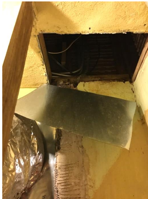
FIGURE 105. Electrical chase panel in the guest room closet.
