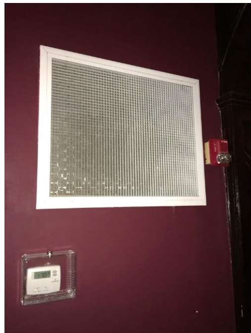
FIGURE 176. Return grille at rear hall.
