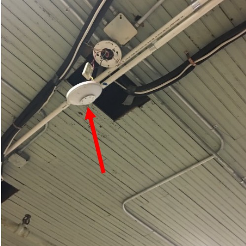
FIGURE 186. Disconnected smoke and fire detectors at basement.
