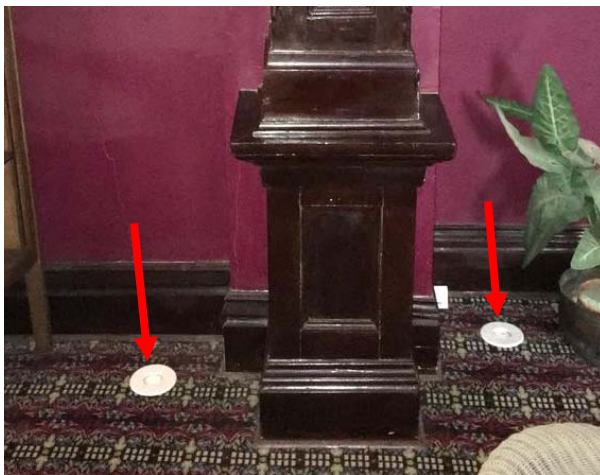
FIGURE 173. Typical Unico distribution nozzle in the carpet floor.
