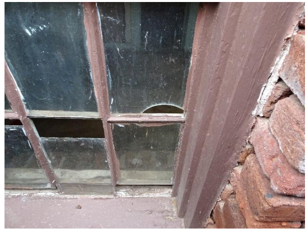
FIGURE 57. Broken and displaced glass at basement windows.
