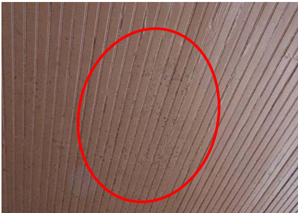
FIGURE 47. Dark spots of biological growth on face of ceiling boards at porch.
