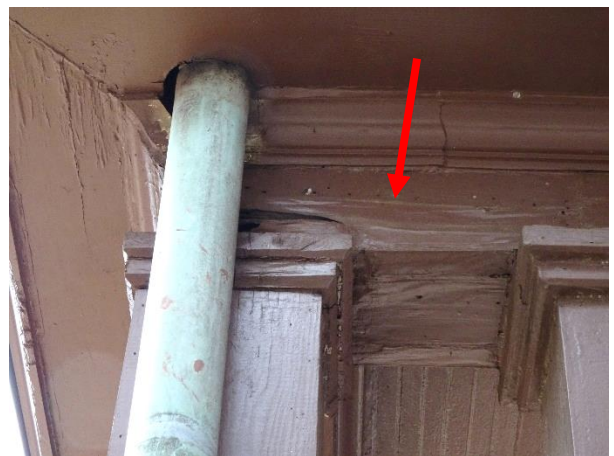
FIGURE 45. Blistering paint at wood porch members.
