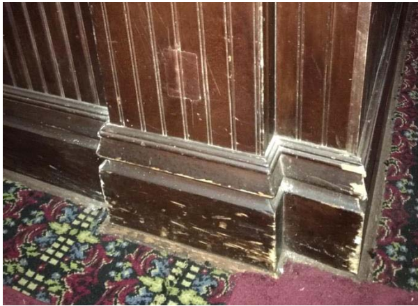
FIGURE 145. General wear and tear at wood base.
