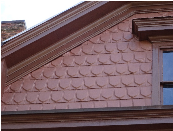
FIGURE 34. Pressed sheet-metal cladding at end gable.
