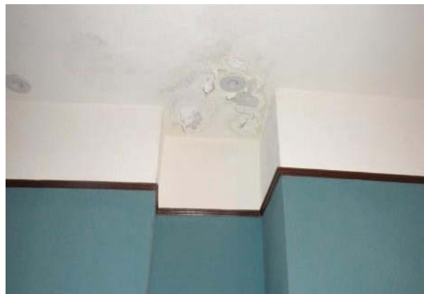
FIGURE 98. Detail of water damage at ceiling, Margaret Washington's bedroom.
