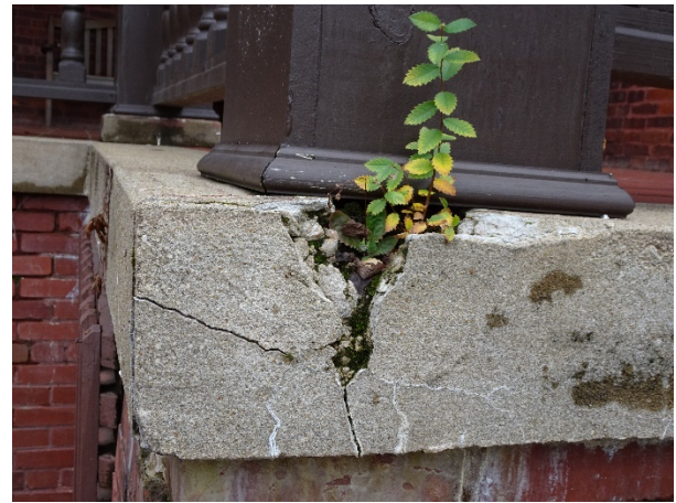
FIGURE 33. Spalling and cracking of concrete at northwest corner of porch.
