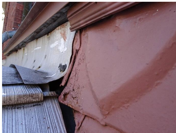
FIGURE 67. Gap at interface between the sheet-metal roof and wall cladding.
