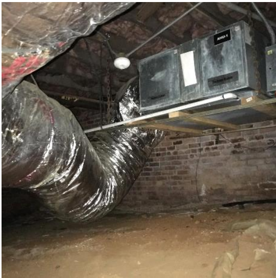
FIGURE 167. Air-handling unit in crawl space.
