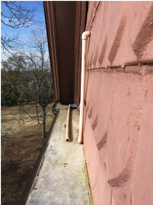
FIGURE 177. Condensate drains from air-handling units and runs on surface of gable infill, spilling into gutter. Pipe disconnected.
