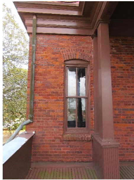
FIGURE 50. Typical masonry window unit showing variation in overall window dimensions and sill extension.
