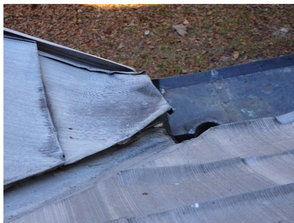
FIGURE 68. Damaged sheet-metal roof cladding near gutter.
