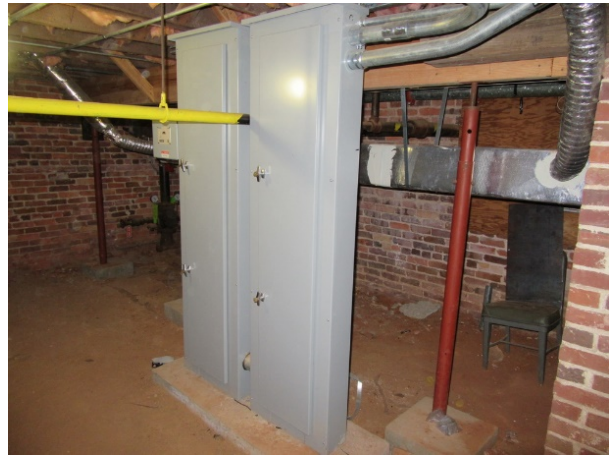
FIGURE 197. Electrical panels at crawl space.
