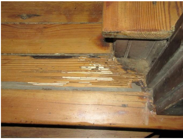
FIGURE 150. Termite damage at basement stair.
