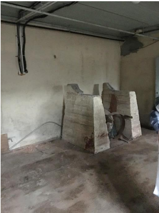
FIGURE 162. Overall view of basement and washtub.
