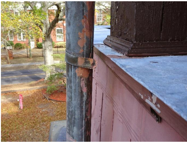
FIGURE 73. Damaged and dislodged downspout strap.
