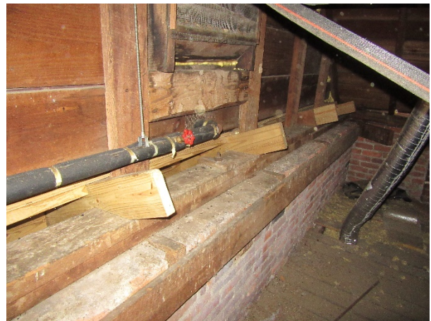
FIGURE 72. Replaced structural kickers at south wing roof.
