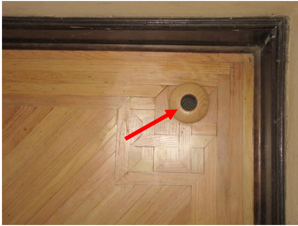
FIGURE 172. Typical Unico distribution nozzle in the parquet floor.
