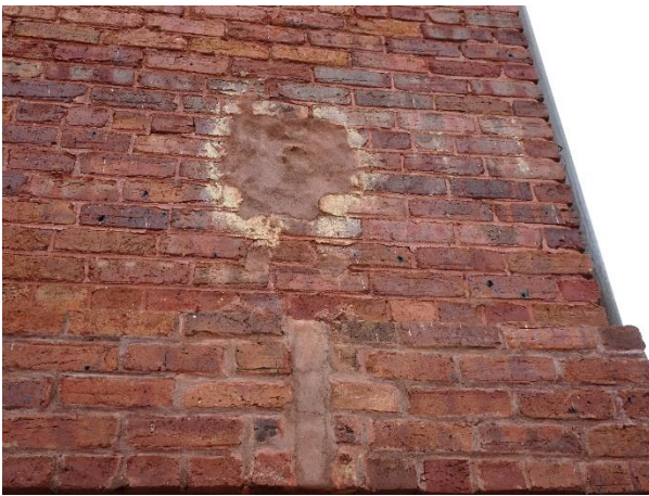
FIGURE 41. Previous cementitious patch repair at abandoned utility openings.
