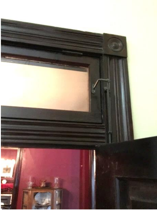
FIGURE 135. Typical door casing with transom.
