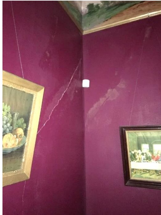
FIGURE 89. Detail of plaster cracking.
