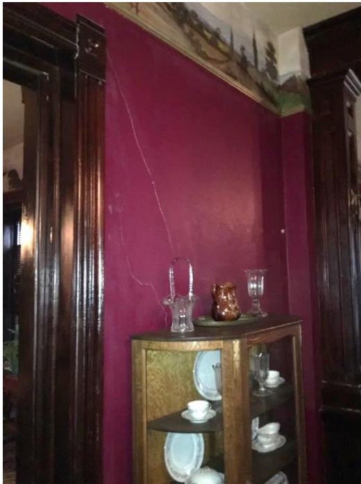
FIGURE 90. Plaster cracking at sliding door pocket (dining room).
