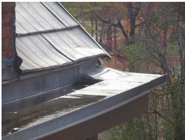
FIGURE 64. Deformed and damaged roofing adjacent to overflowing gutter.
