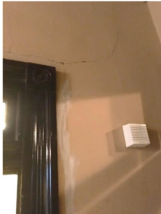
FIGURE 93. Detail of plaster cracking at sides of door frame.
