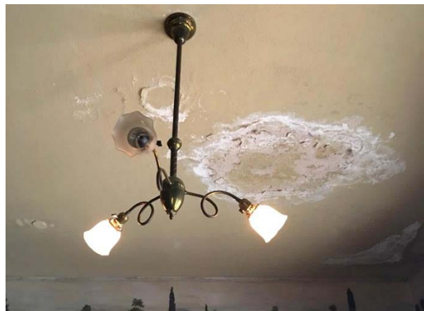
FIGURE 97. Detail of plaster damage at ceiling.
