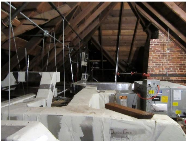
FIGURE 168. Air-handling unit at attic.
