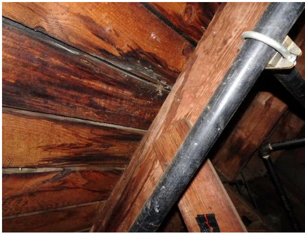
FIGURE 70. Moisture staining at wood sheathing.
