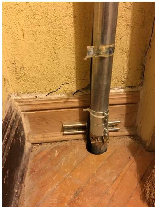
FIGURE 106. Conduit penetration in the guest room closet floor.
