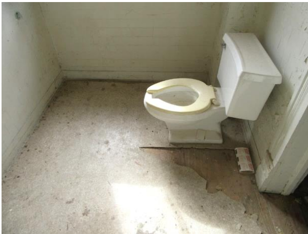
FIGURE 132. Deteriorated linoleum floor in the third-floor bathroom.
