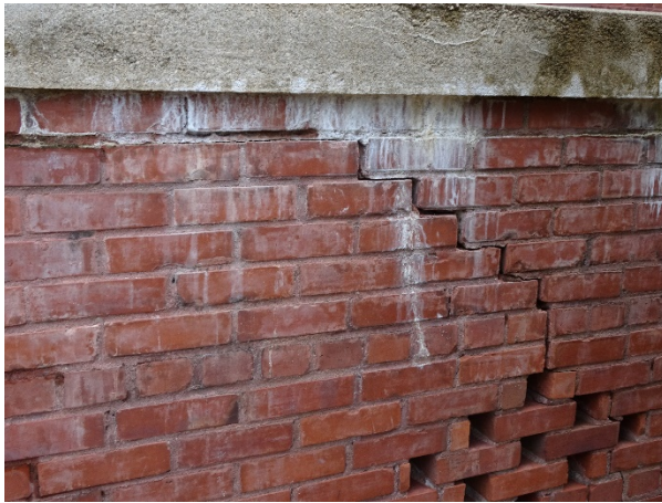
FIGURE 24. Step cracking and efflorescence at the porch walls.
