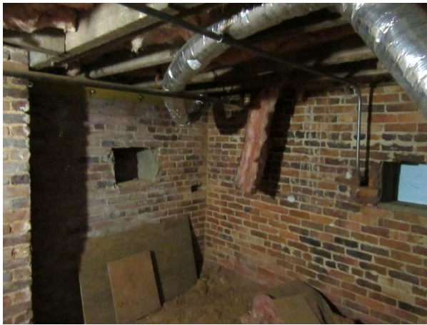
FIGURE 163. Mechanical crawl space / basement, insulation displaced at floor joists.
