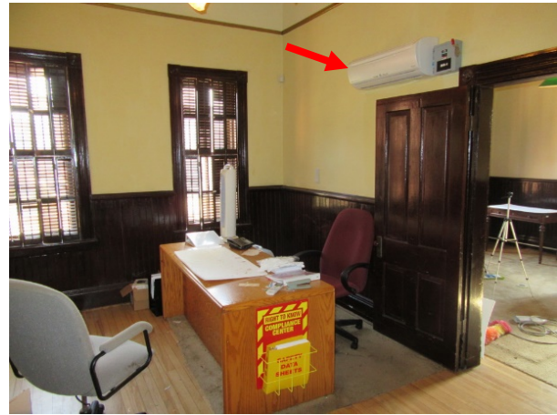
FIGURE 170. Wall-mounted VRF unit at breakfast room.
