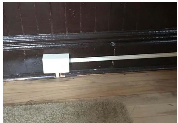
FIGURE 203. Detail of surface-applied conduit at floor penetration.
