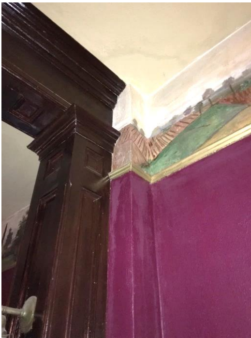
FIGURE 94. Paint damage at dining room addition.
