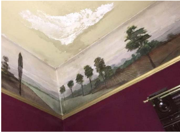
FIGURE 113. Frieze mural at dining room addition, affected by water staining.
