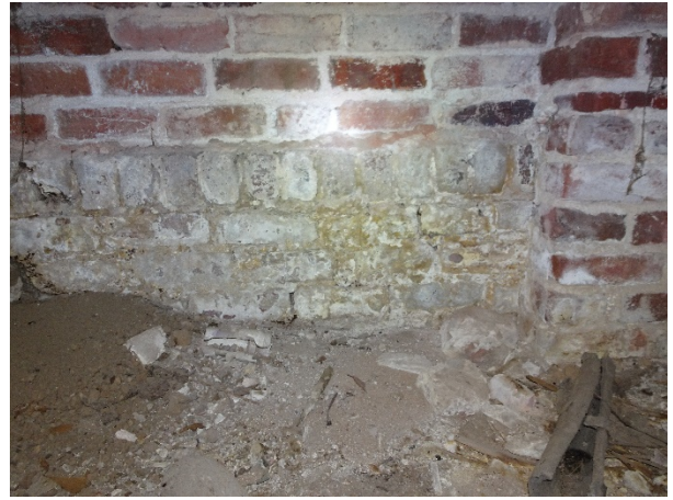
FIGURE 26. Accumulation of efflorescence at base courses of the porch walls.
