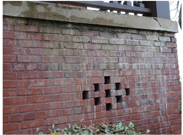
FIGURE 27. Moisture staining at porch walls.
