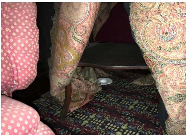
FIGURE 174. HVAC distribution nozzle located below furniture and table cloth.
