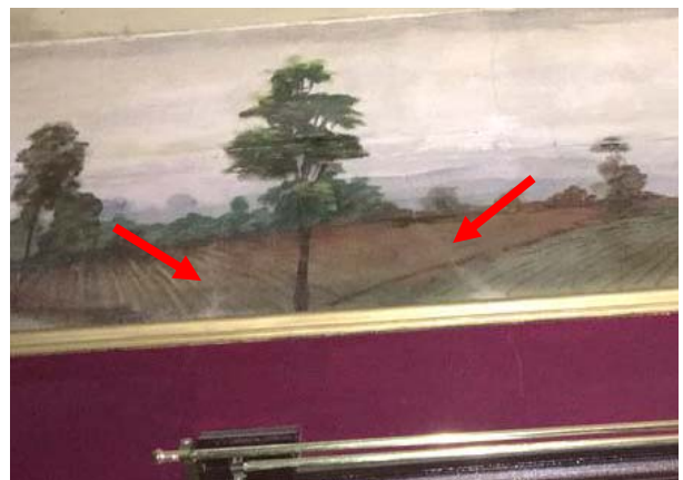
FIGURE 116. Previously repaired crack at mural where retouched paint is visible.
