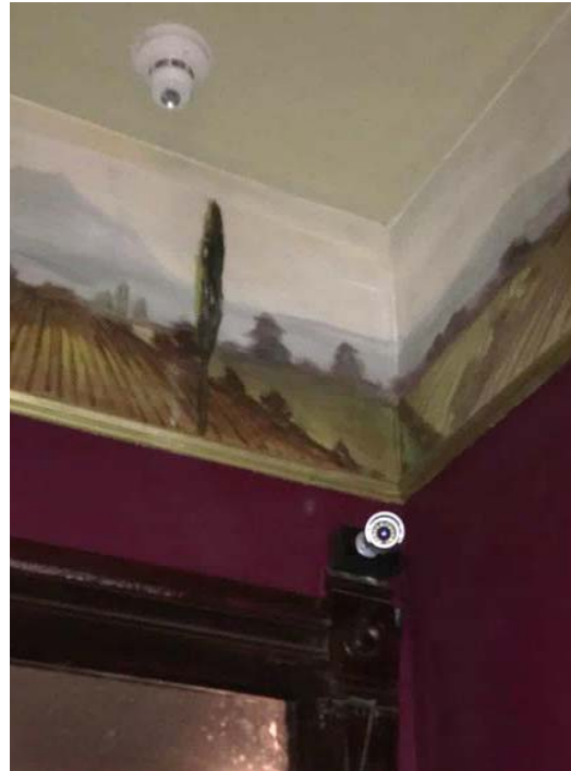
FIGURE 180. Smoke detector and security camera at dining room.
