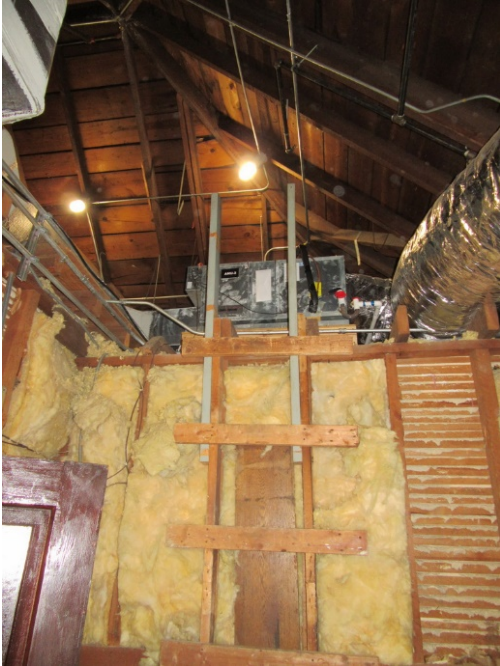
FIGURE 161. Missing insulation at attic side of third-floor wall.
