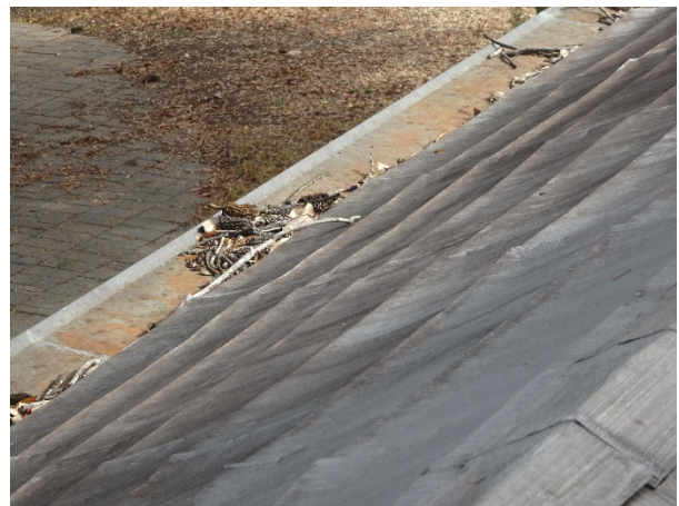
FIGURE 62. Debris and organic matter block a gutter.
