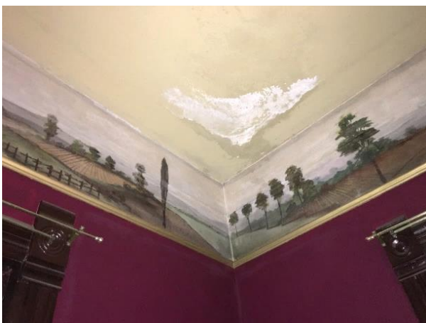
FIGURE 96. Water damage at ceiling.
