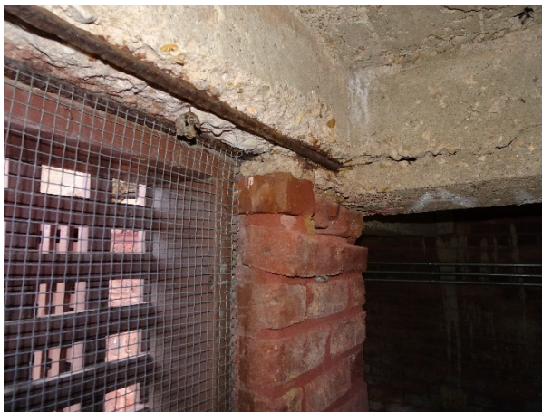
FIGURE 31. Spalled concrete bond beam at porch wall.
