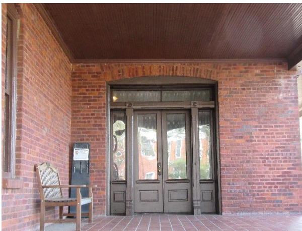
FIGURE 52. Main entrance door on the north elevation.
