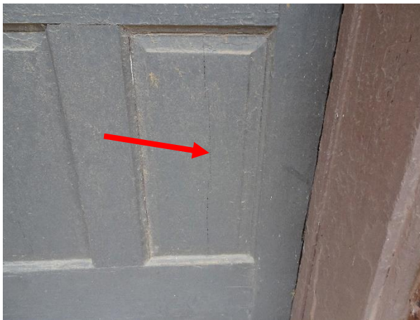
FIGURE 55. Vertical crack in recessed panel.
