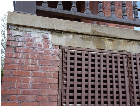
FIGURE 32. Moisture staining and evidence of moisture infiltration at concrete bond beam.
