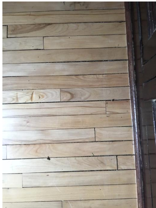
FIGURE 126. Separations at wood floor in pantry.
