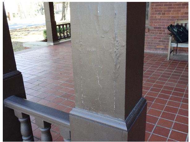
FIGURE 44. Debonded paint and plaster coating at columns.
