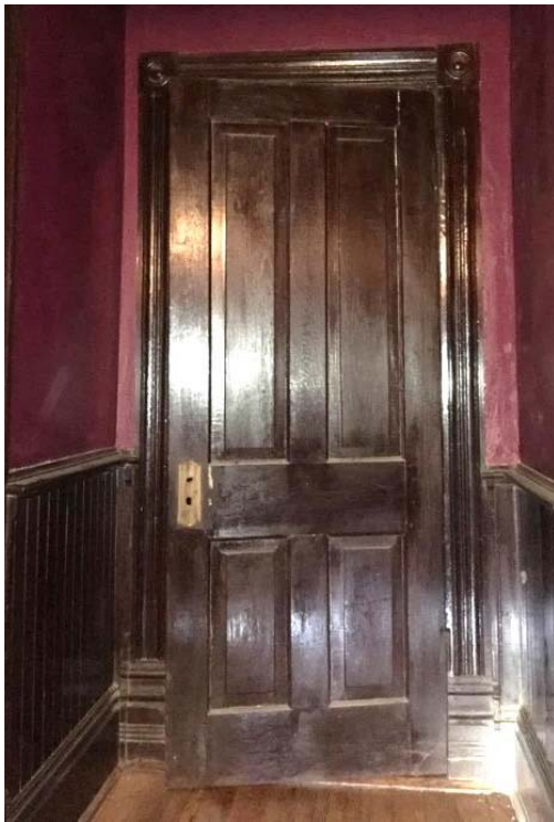
FIGURE 158. Door at rear stair, hardware missing.
