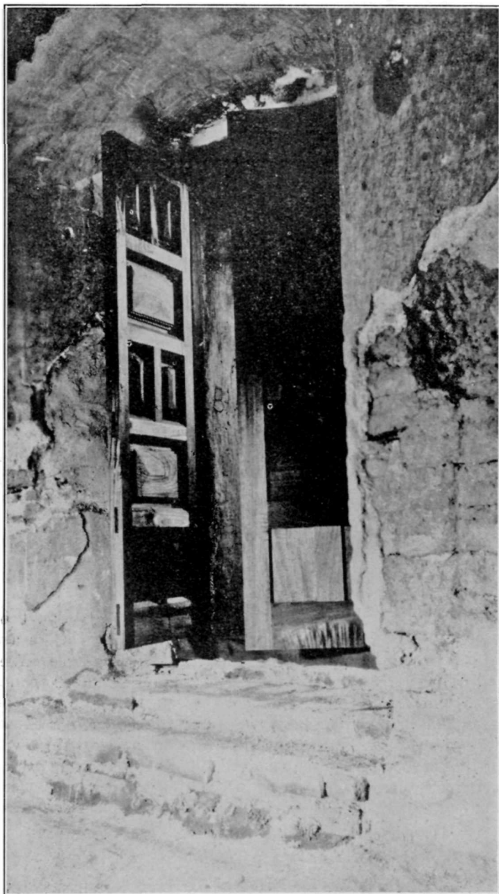
Sacristy doorway from the Sanctuary side.
