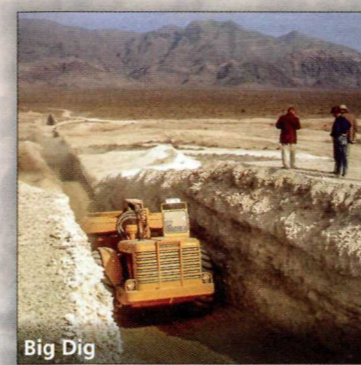
Big Dig NEVADA STATE MUSEUM, CARSON CITY
