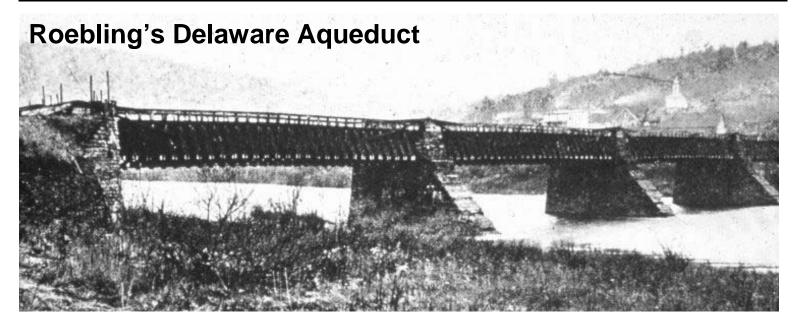
Upper Delaware Scenic and Recreational River is the home of the oldest existing wire cable suspension bridge in the nation — the Delaware Aqueduct, or Roebling Bridge as it is now known. Begun in 1847 as one of four suspension aqueducts on the Delaware and Hudson Canal, it was designed by and built under the supervision of John A. Roebling, future engineer of the Brooklyn Bridge.
