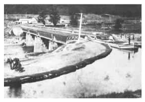
The aqueduct operated for fifty years until the closing of the canal in 1898. It was then converted to a private toll bridge and underwent a series of modifications through the years. Around 1900, new owner Charles Spruks built a tollhouse abutting the New York side of the structure.
