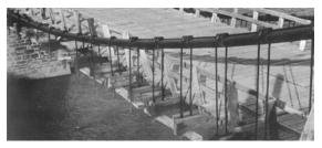
Each 8 1/2-inch diameter suspension cable carries 2,150 wires bunched into seven strands. Laboratory tests in 1983 concluded that the cable was still "viable;" some of the wires even exceeded Roebling's original specifications. Roebling's cast iron "pier
