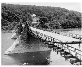
When the National Park Service started restoration work, the primary goal was to preserve the structural integrity of the bridge and as much of the original ironwork as possible. Almost all of the Delaware Aqueduct's existing ironwork — cables, saddles, and suspenders — are the same materials installed when the structure was built. The two suspension cables are made of wrought iron strands, spun on site under the direction of John Roebling in 1847.
