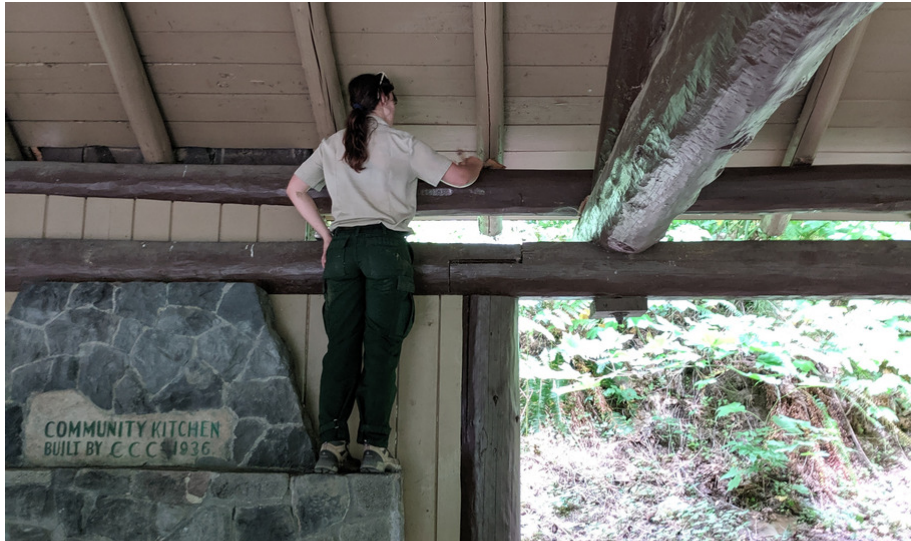
Painting the roof on the Eagle Creek Community Kitchen
