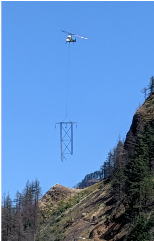
Helicopter removing an old transmission tower
