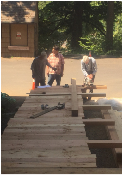
A new bridge being built for Eagle Creek Trail
